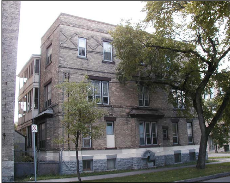
Rear (north) and west façades, 2002
