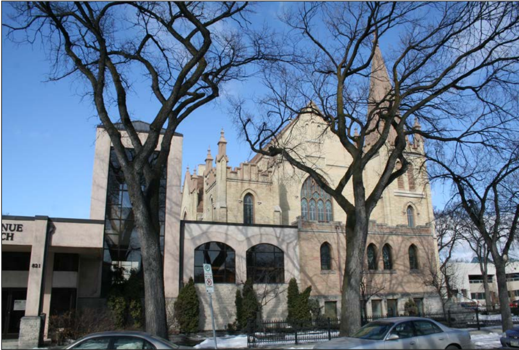
South façade and portion of west addition, 2009
