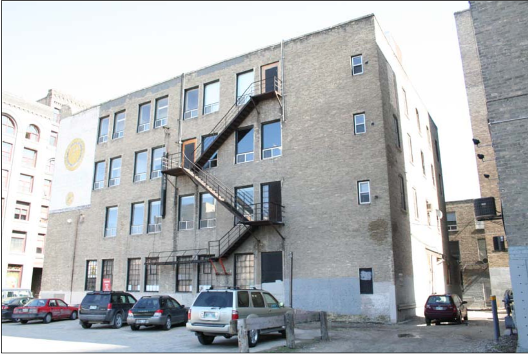
Plate 9 – Merchants Building, 250 McDermot Avenue, rear (south) façade. (M. Peterson, 2007.)
