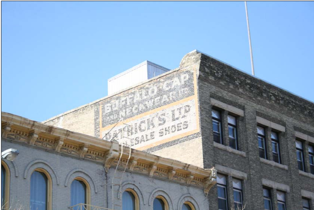
Plate 10 – Merchants Building, 250 McDermot Avenue, northeast corner. (M. Peterson, 2007.)
