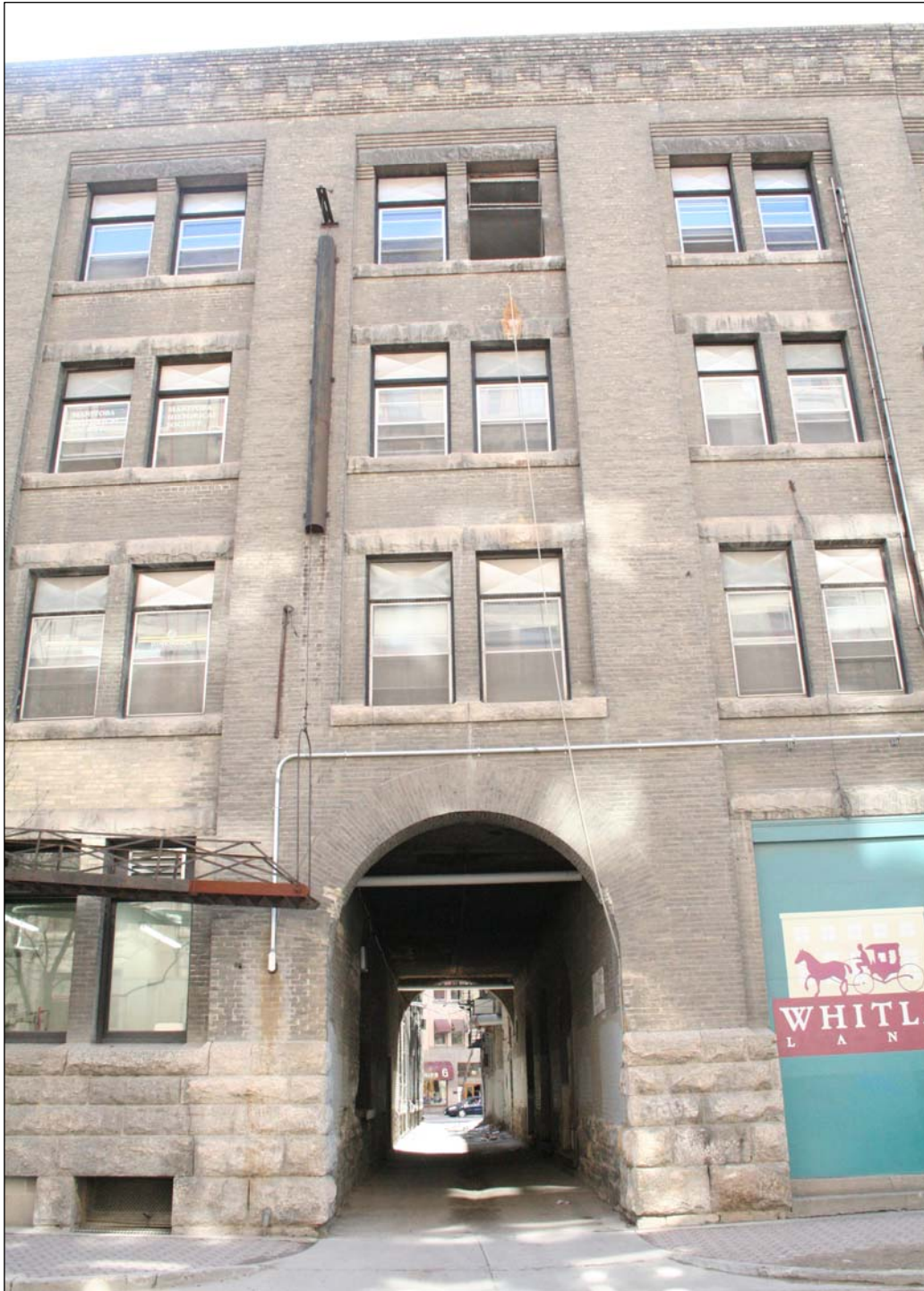
Plate 7 – Merchants Building, 250 McDermot Avenue, dray way entrance, west side. ( M. Peterson, 2007. )
