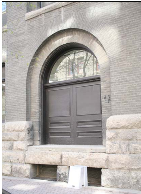
Plate 6 – Merchants Building, 250 McDermot Avenue, west façade loading doors. ( M. Peterson, 2007. )
