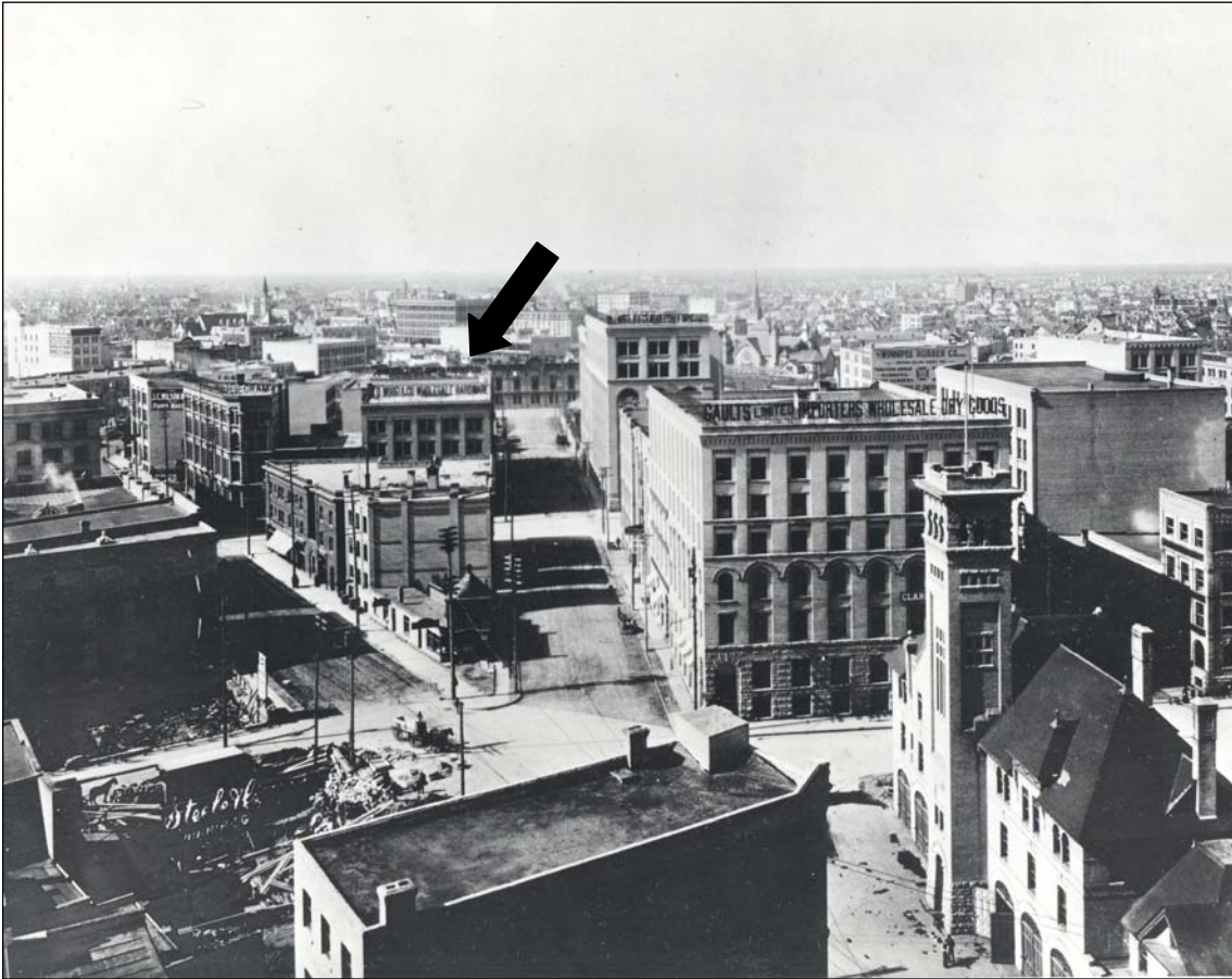
Plate 1 – Looking south along Arthur Street from Bannatyne Avenue into the heart of Winnipeg’s Exchange District west of Main Street, ca.1905, including the George D. Wood & Company Building (arrow). ( Courtesy of the Archives of Manitoba, Winnipeg-Views c1905- 2. )
