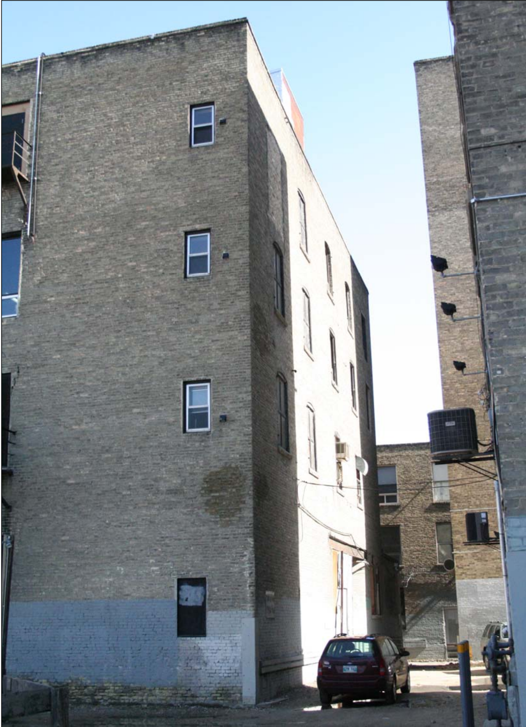
Plate 12 – Merchants Building, 250 McDermot Avenue, east façade, south end. ( M. Peterson, 2007. )
