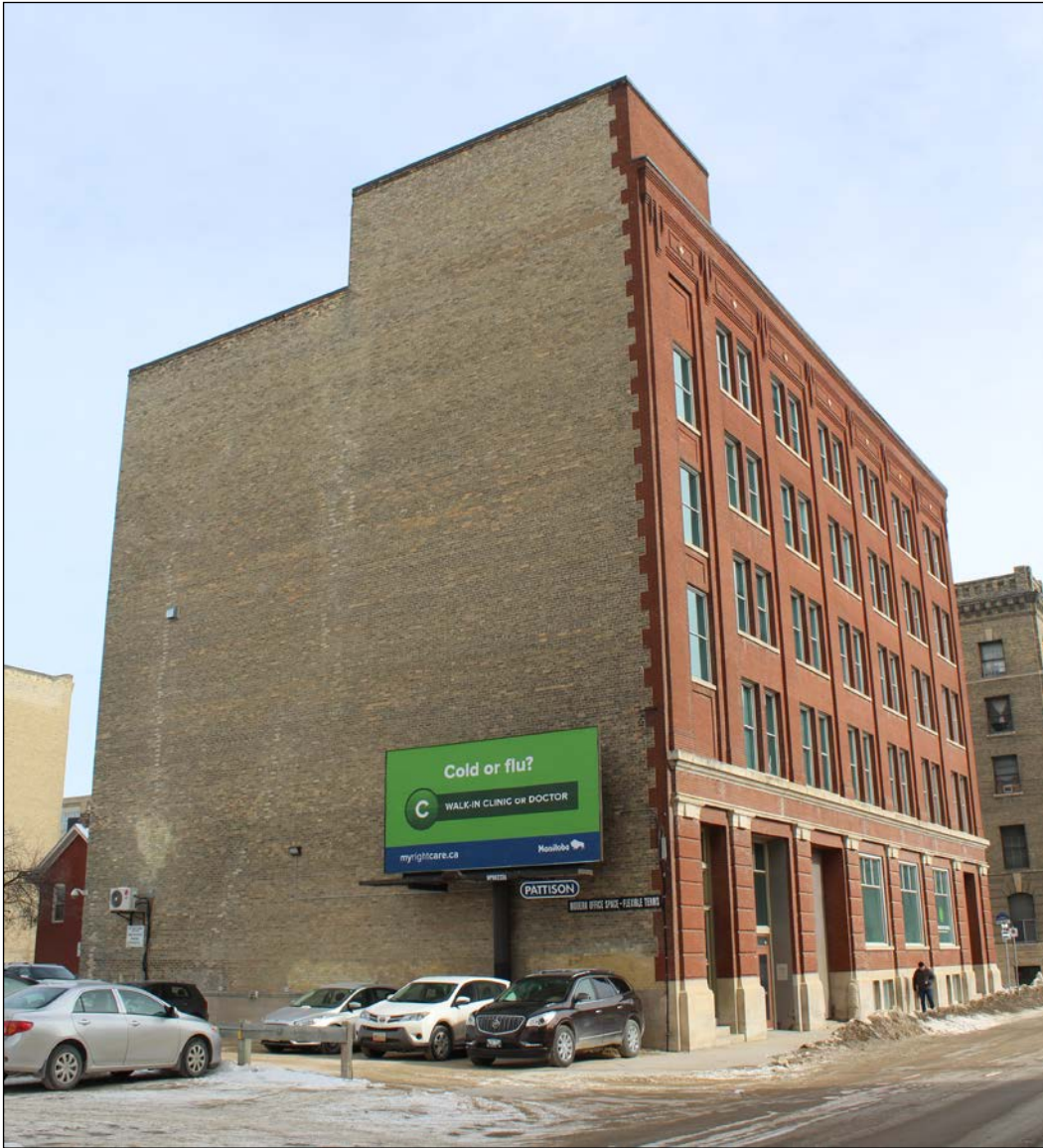
Plate 14 – Western Glove Building (Former Finnie and Murray Block), 321 McDermot Avenue, south and west façades, 2023. (M. Peterson, 2023.)
