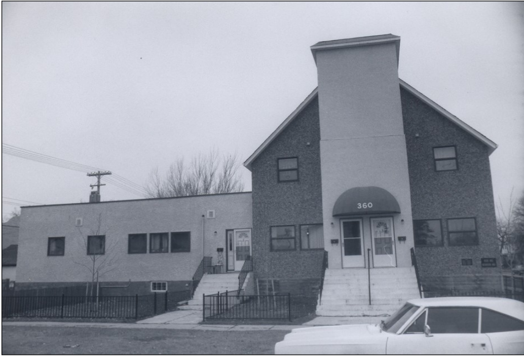
Front (east) façade detail, 1978
