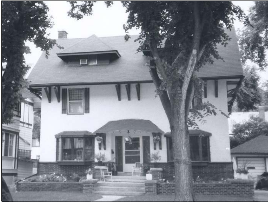
Front (east) façade detail, 1978
