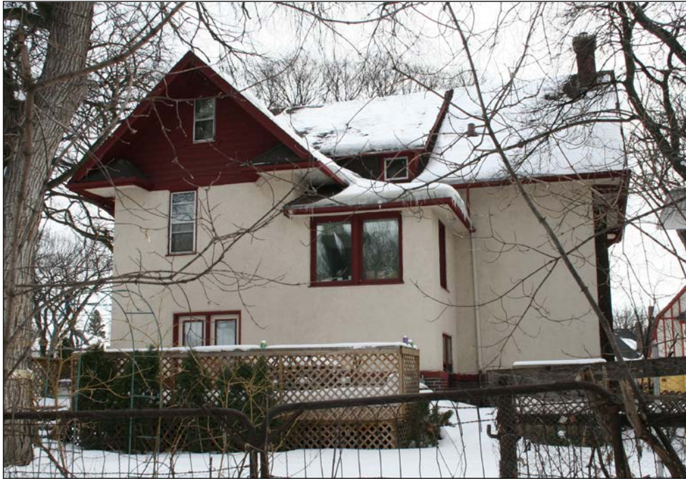
Rear (west) façade, 2009
