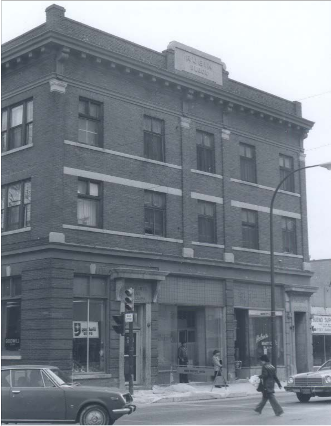
Plate 12 – Rubin Block/Morley Apartments, 270 Morley Avenue, west façade with original recessed entrances and prism lights, ca.1980. (M. Peterson, 2017.)
