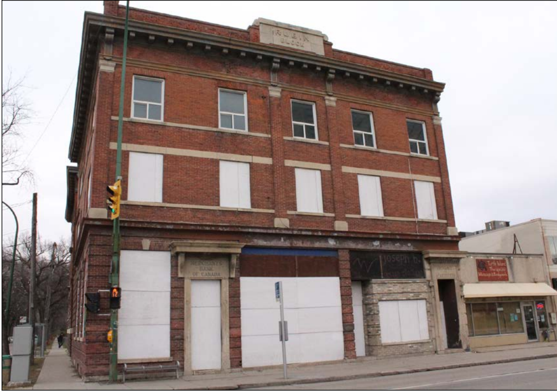
Plate 6 – Rubin Block/Morley Apartments, 270 Morley Avenue, 2017. (M. Peterson, 2017.)
