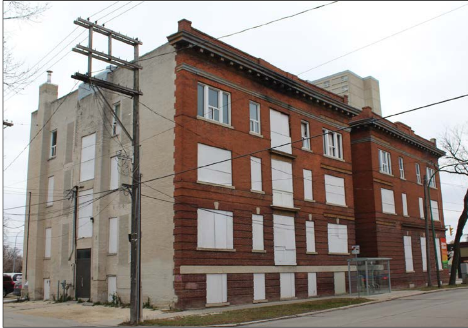
Plate 10 – Rubin Block/Morley Apartments, 270 Morley Avenue, east and north façades, 2017. ( M. Peterson, 2017. )
