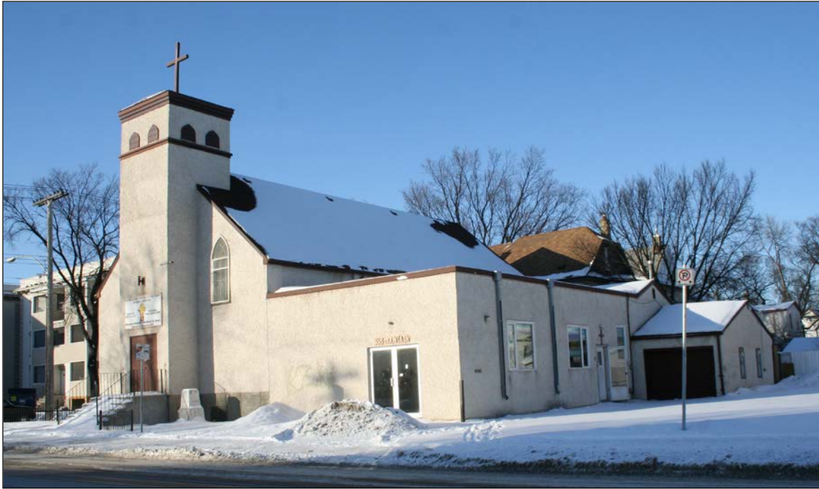
Front (south) and east façades, 2009
