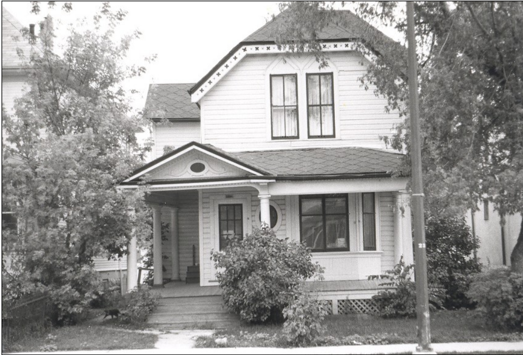
Front (south) façade, 1978
