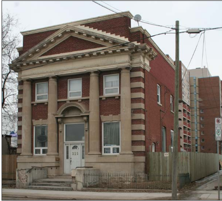
Front (south) and east façades, 2009
