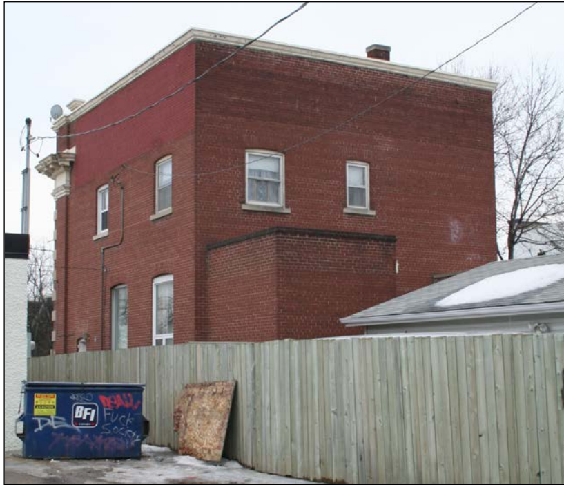
Rear (north) and east façades, 2009
