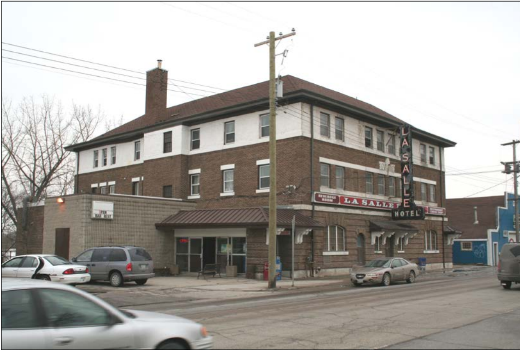
Front (north) and west façades, 2009
