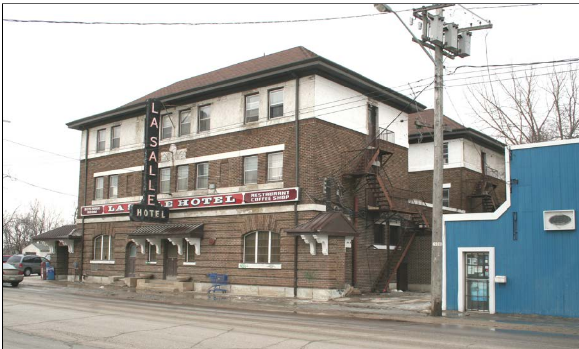
Front (north) and west façades, 2009
