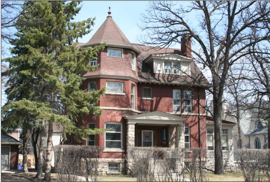
Front (west) and north façades, 2009
