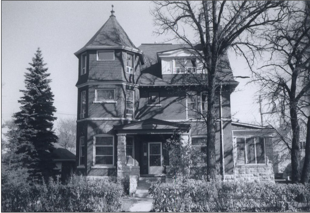
Front (west) façade, 1978
