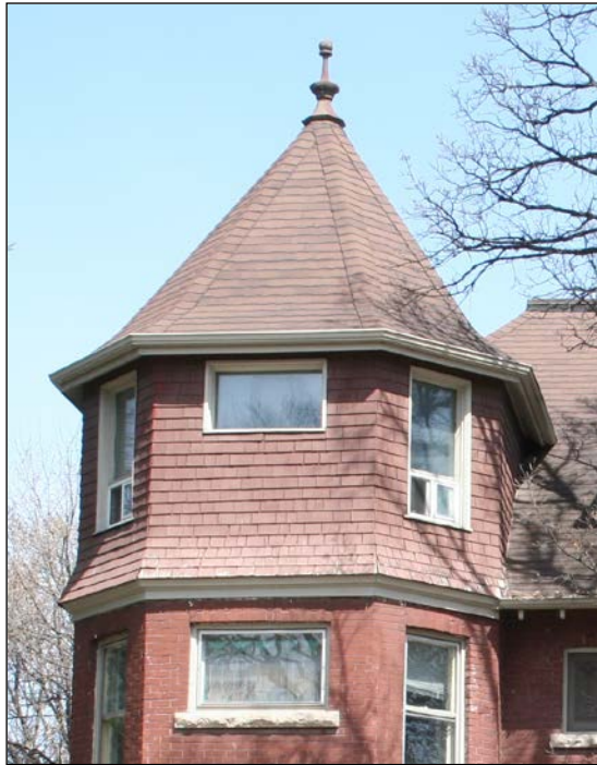
Front (west) façade detail, 2009
