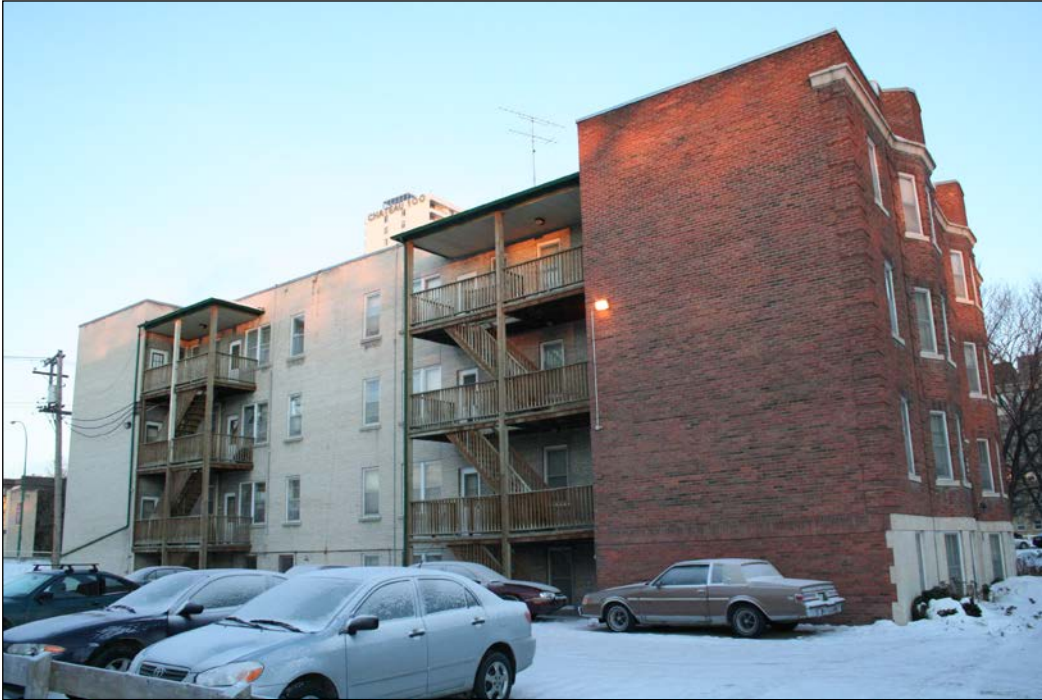
Front (east) and south façade, 2008
