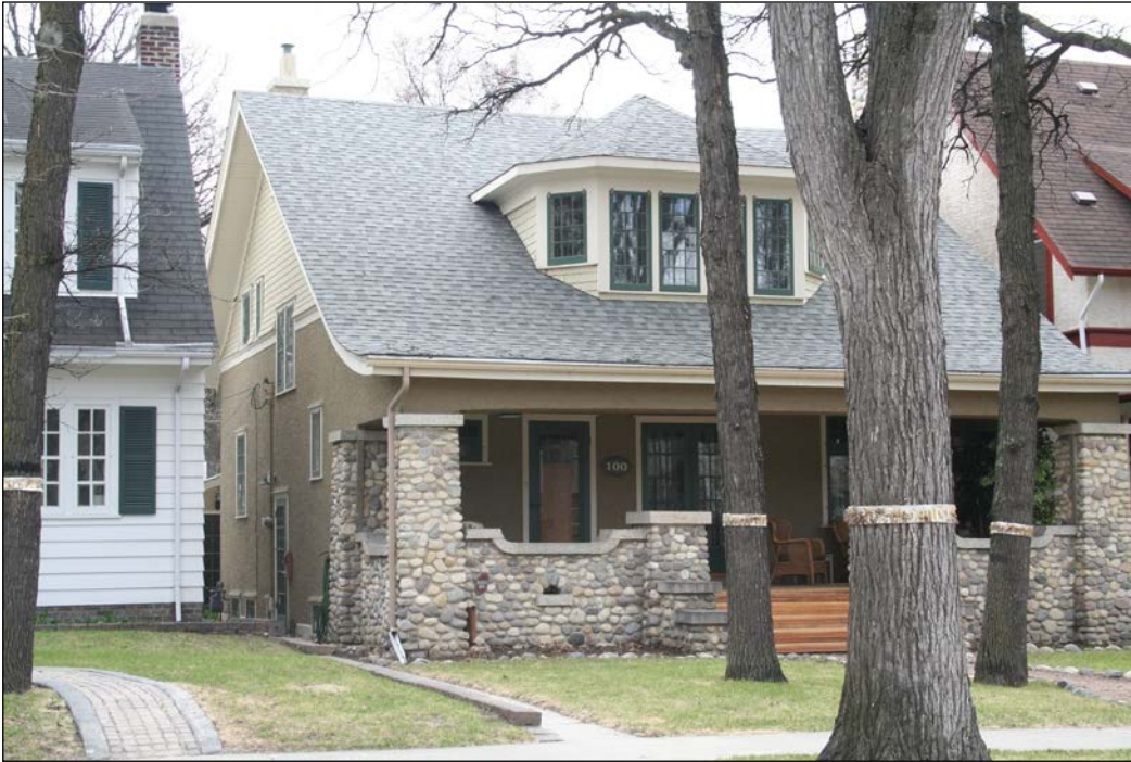
Front (west) and north façades, 2009
