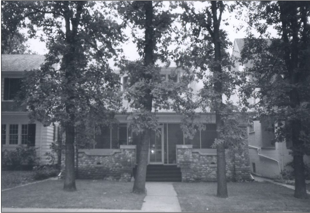
Front (west) façade, 1978
