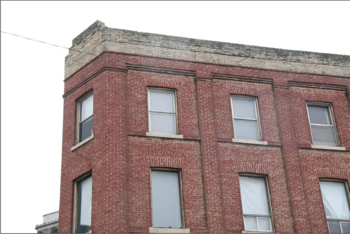
Plate 8 – Oxford Hotel, 216 Notre Dame Avenue, detail of roofline, 2015. (M. Peterson, 2015.)
