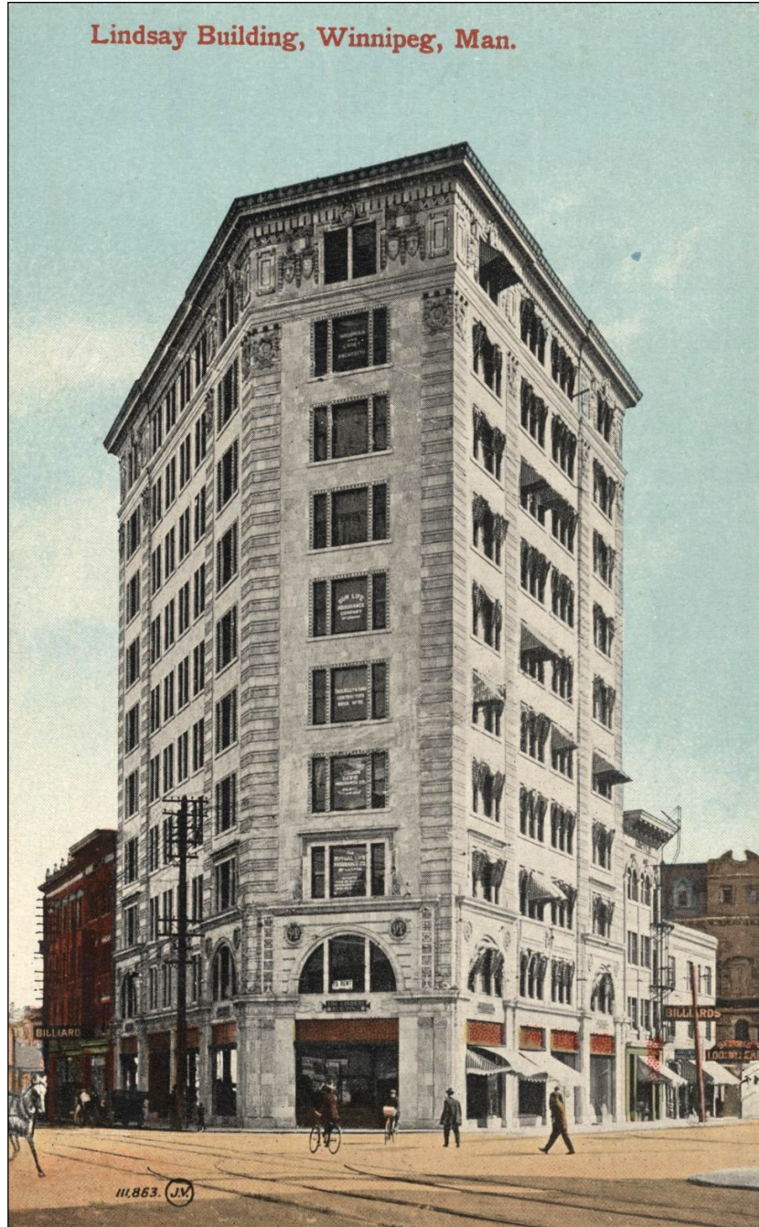
Plate 15 – Lindsay Building, 228 Notre Dame Avenue, no date. (City of Winnipeg.)
