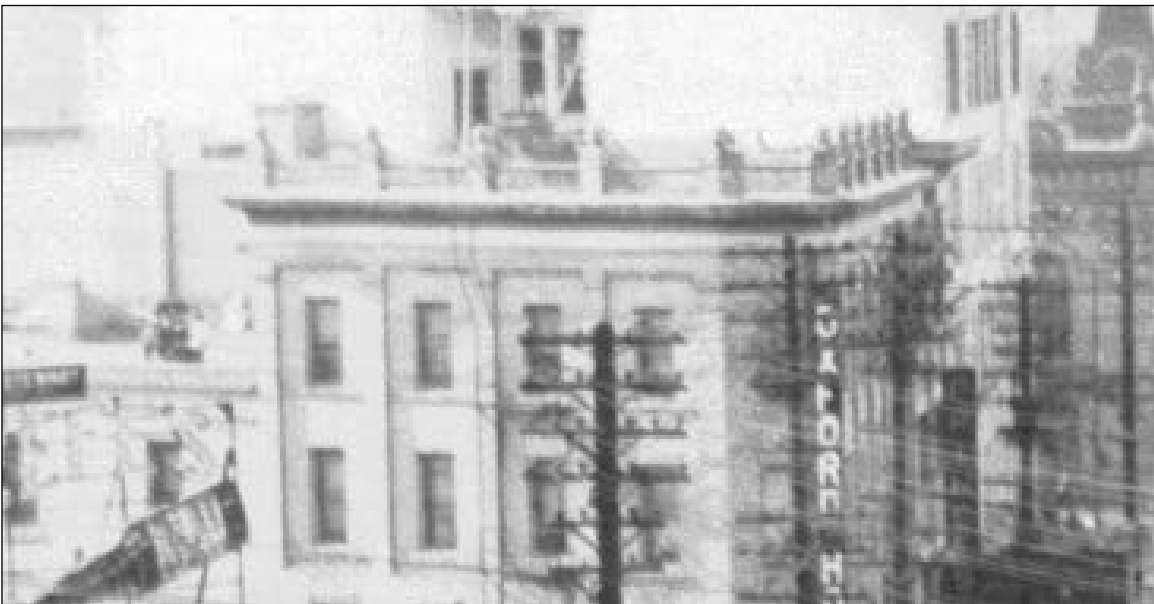
Plate 9 – Detail of original Oxford Hotel roofline, 1911, which included cornice and ornate parapet. (Courtesy of the Archives of Manitoba.)
