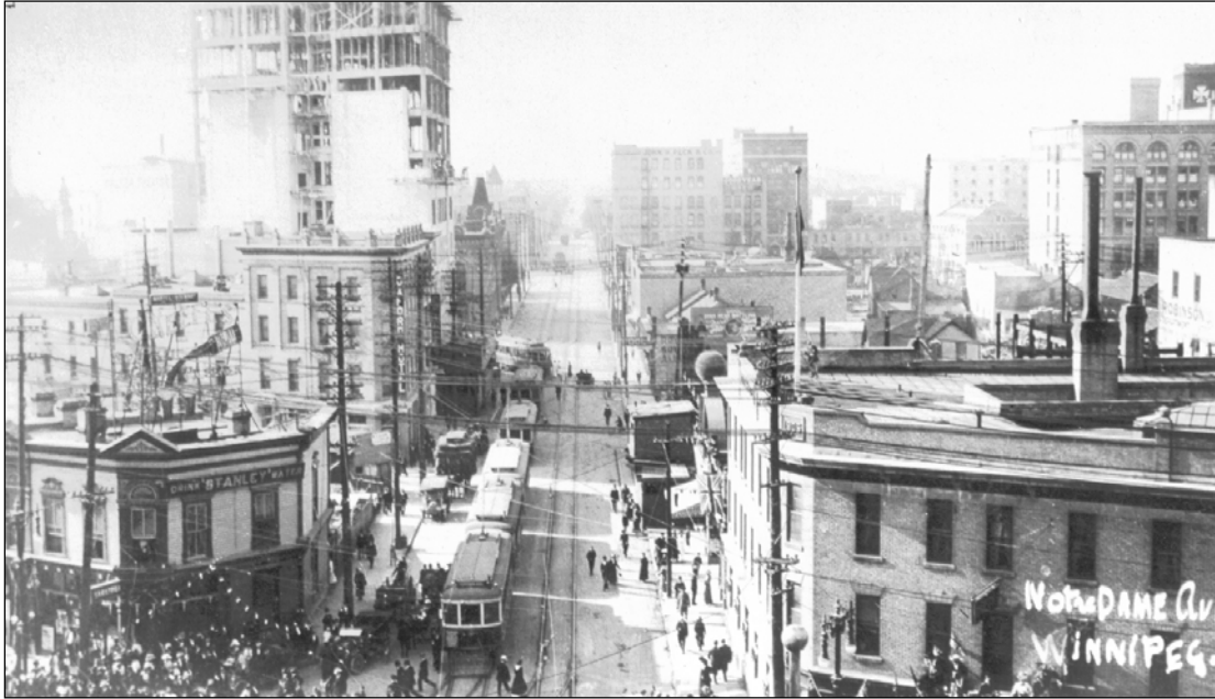
Plate 4 – Notre Dame Avenue, 1911. Construction is well underway on the Lindsay Building, but has not yet started on the Electric Railway Chambers. (Courtesy of the Provincial Archives of Manitoba.)
