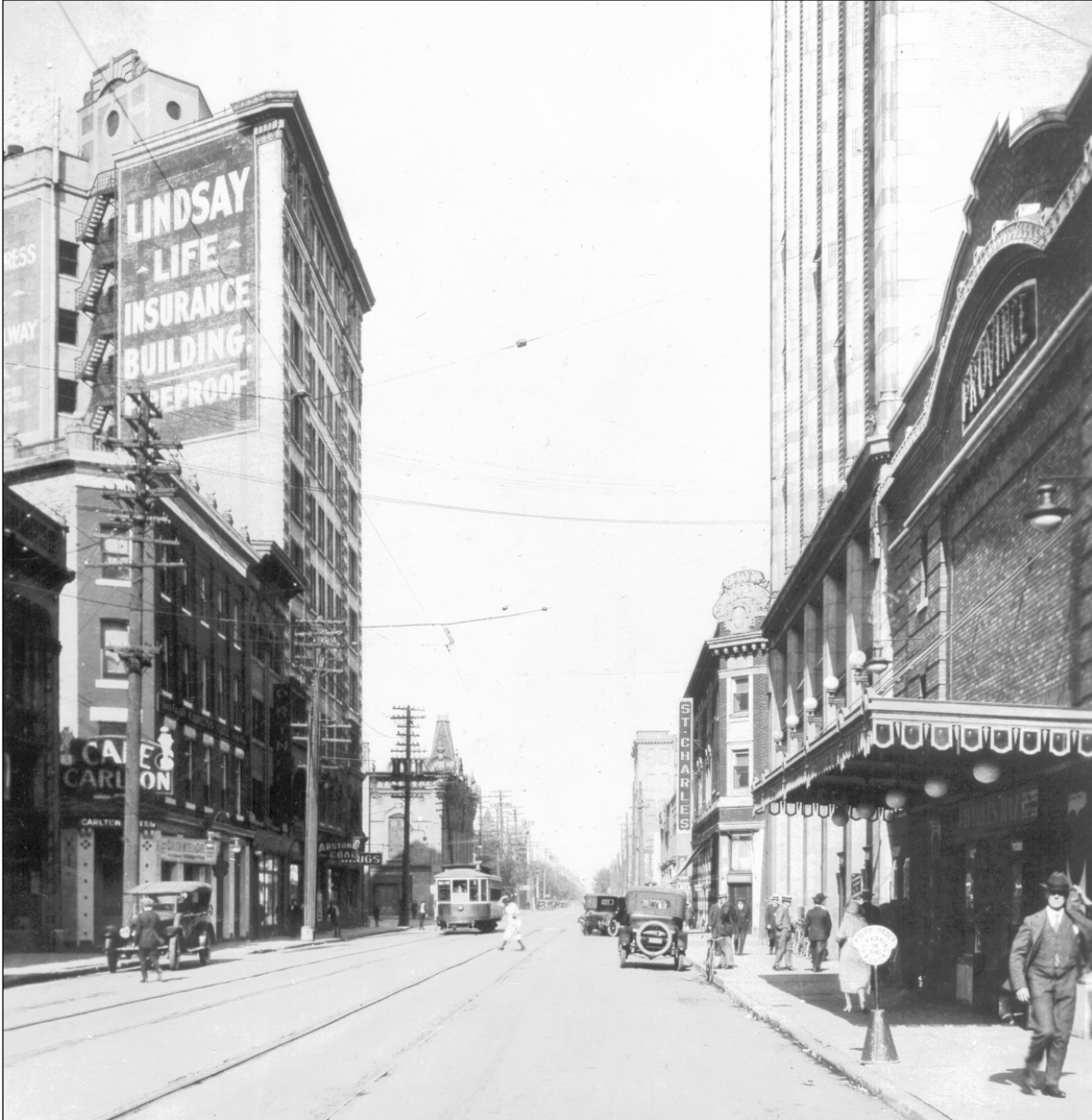
Plate 2 – Looking north on Notre Dame Avenue, ca.1927. To the left is the Oxford Hotel, the Princess (Argyle) Block, the Lindsay Building with Grace Methodist in the background. On the right are the Province Theatre, the Winnipeg Electric Railway Chambers and the St. Charles Hotel. (Courtesy of the Provincial Archives of Manitoba.)
