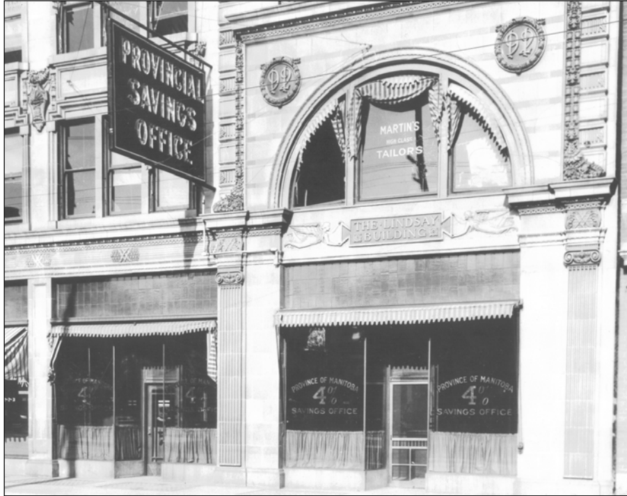
Plate 5 – The Provincial Savings Office in the Garry Street side of the Lindsay Building, ca.1925. This shot details the original features of the ground floor. (Courtesy of the Provincial Archives of Manitoba. )
