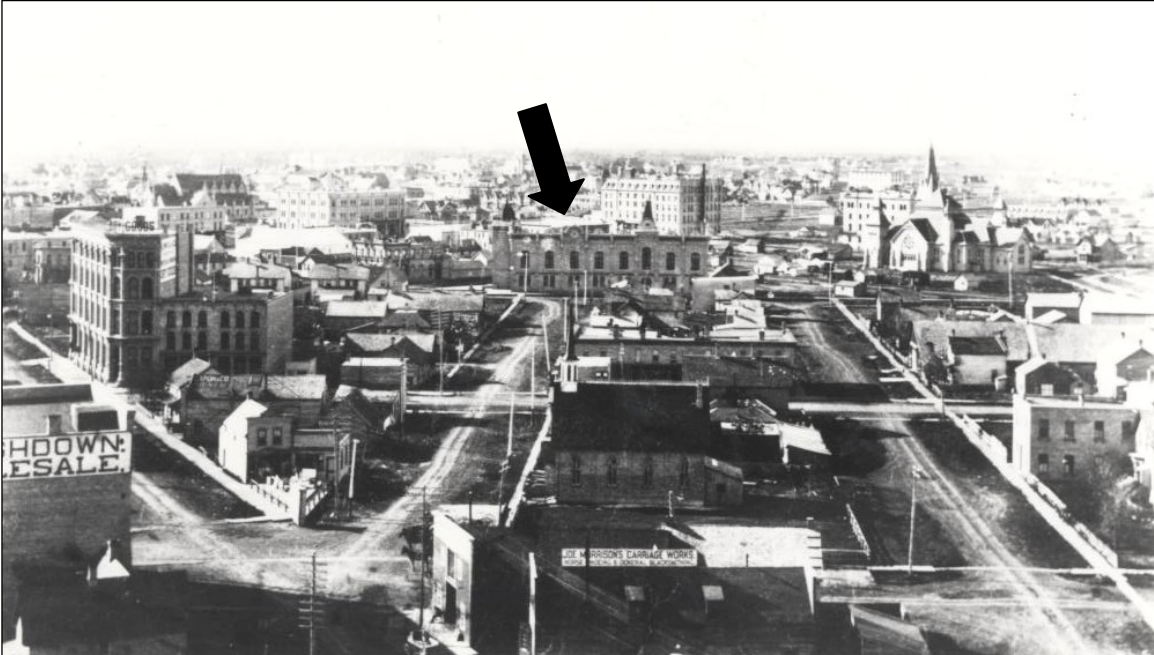
Plate 5 – Looking south from City Hall, ca.1887. Grace Methodist Church (arrow), which was located across Notre Dame Avenue from the Christie Block, dominated the area and was a fitting neighbour to Knox Presbyterian to the right. ( Archives of Manitoba. )
