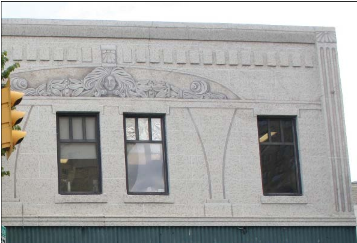
Plate 13 – Christie Block, 245 Notre Dame Avenue, detail of second floor renovations, 2014. (M. Peterson, 2014.)
