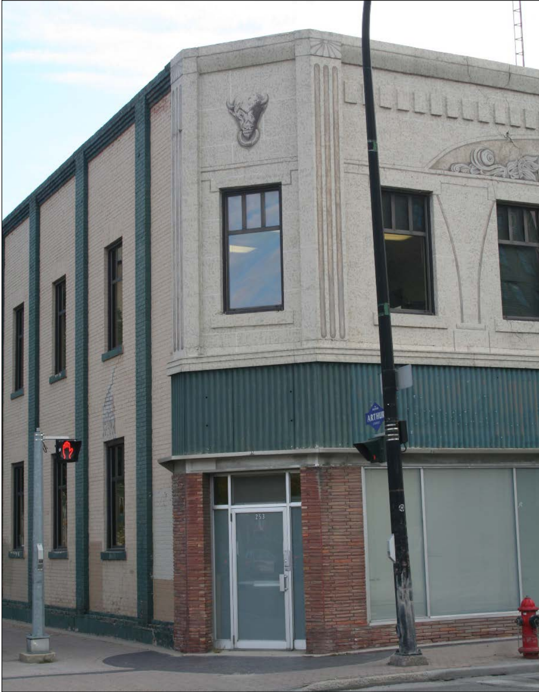
Plate 15 – Christie Block, 245 Notre Dame Avenue, southwest corner, 2014. (M. Peterson, 2014.)
