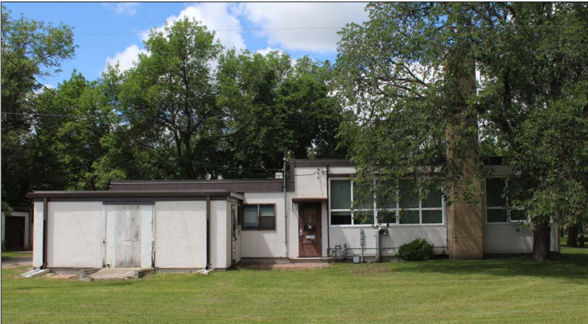
Plate 17 – Brookside Cemetery, Administration Building, 3001 Notre Dame Avenue, rear (east) façade, 2021. (M. Peterson, 2021.)
