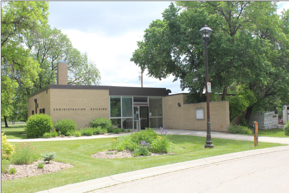
Plate 14 – Brookside Cemetery, Administration Building, 3001 Notre Dame Avenue, front (west) façade, 2021. ( M. Peterson, 2021. )
