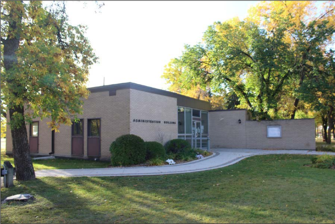
Plate 10 – Brookside Cemetery Administration Building, 3001 Notre Dame Avenue, 2020. ( M. Peterson, 2020. )
