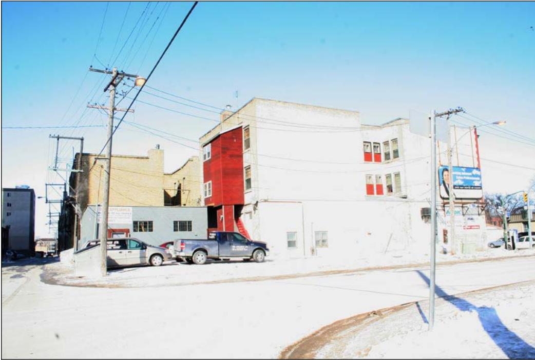
Rear (south) and east façades, 2009
