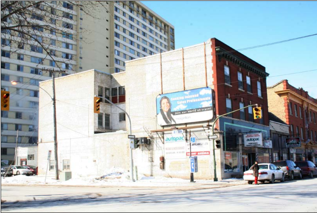
Front (north) and east façades, 2009
