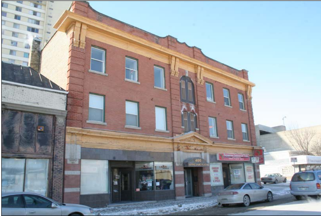
Front (north) and east façades, 2009
