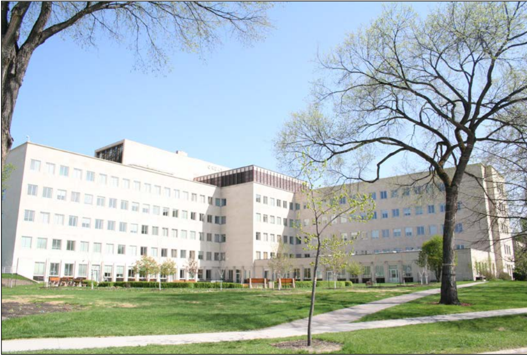
Rear (west) and north façades, 2007
