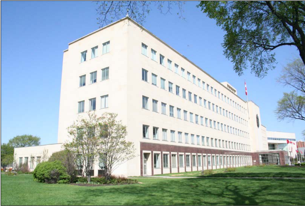
Front (east) and south façades, 2007
