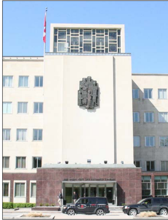
Detail of main (east) entrance, 2007
