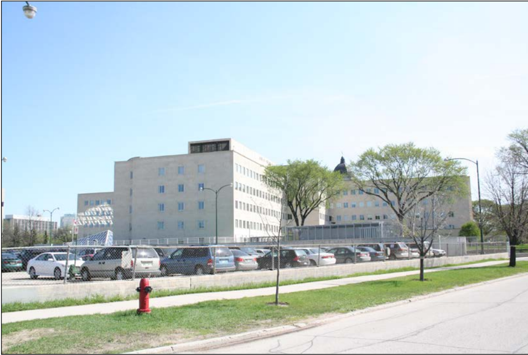
Rear (west) and south façades, 1994
