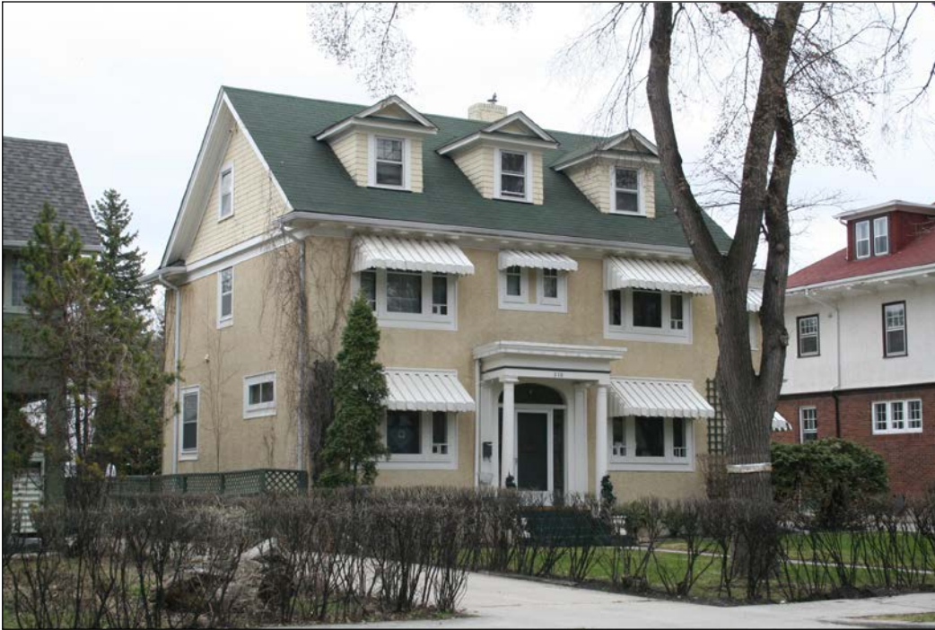
Front (west) and north façades, 2009
