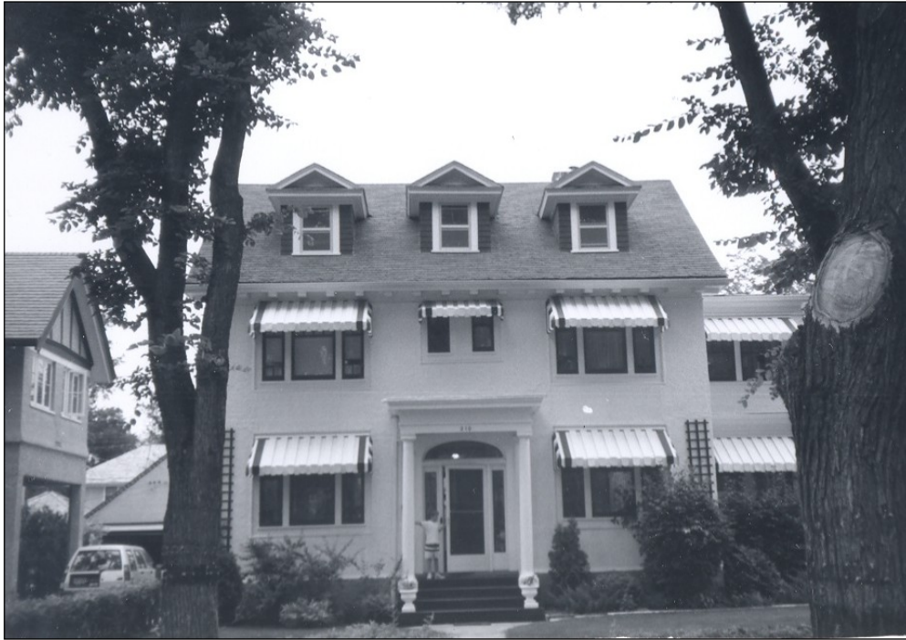
Front (west) façade, 1978
