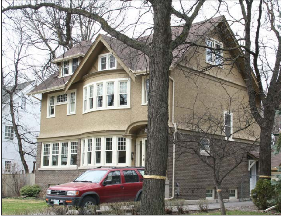
Front (east) and north façades, 2009
