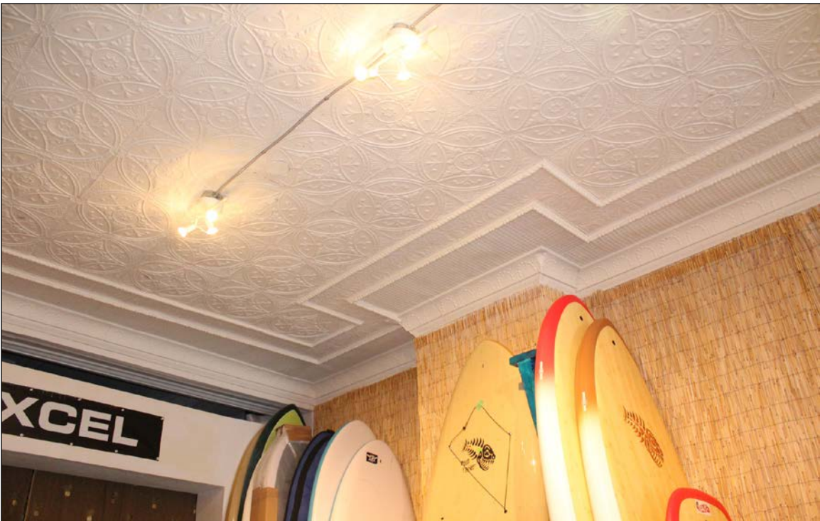
Plate 18 – Johnstone Block (Kuo Min Tang Building), 209 Pacific Avenue, tin ceiling, #209 Pacific Avenue,, 2019. ( M. Peterson, 2019. )
