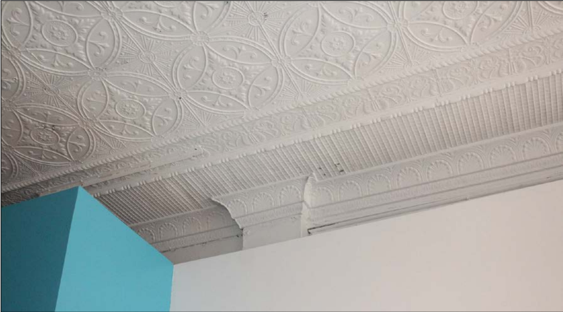
Plate 17 – Johnstone Block (Kuo Min Tang Building), 209 Pacific Avenue, tin ceiling, #211 Pacific Avenue, 2019. ( M. Peterson, 2019. )
