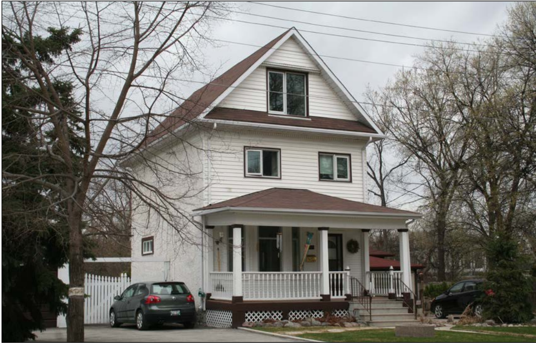
Front (north) and east façades, 2009
