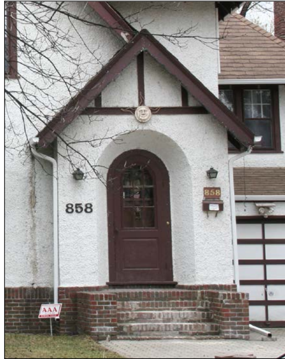
Front (north) façade detail, 2009
