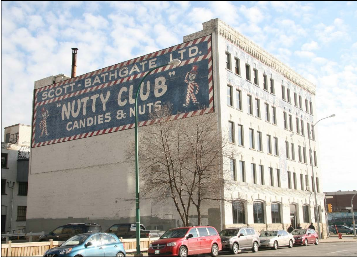
Plate 9 – Scott-Bathgate Building, 149 Pioneer Avenue, front (south) and west façades, 2015. (M. Peterson, 2015.)
