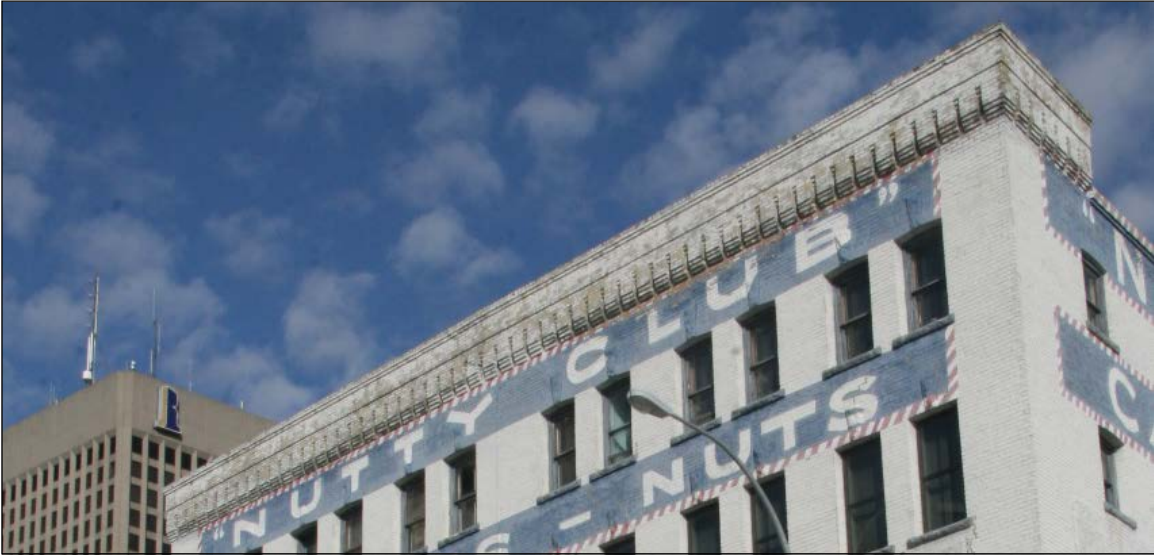
Plate 7 – Scott-Bathgate Building, 149 Pioneer Avenue, detail of front (south) cornice, 2015. (M. Peterson, 2015.)
