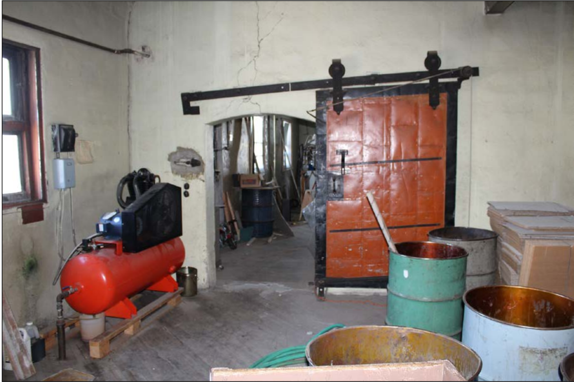
Plate 14 – Scott-Bathgate Building, 149 Pioneer Avenue, 5 th floor connecting doorway with metal-clad fire door, 2017. ( M. Peterson, 2017. )
