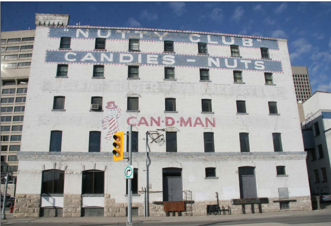
Plate 8 – Scott-Bathgate Building, 149 Pioneer Avenue, east façade, 2015. (M. Peterson, 2015.)
