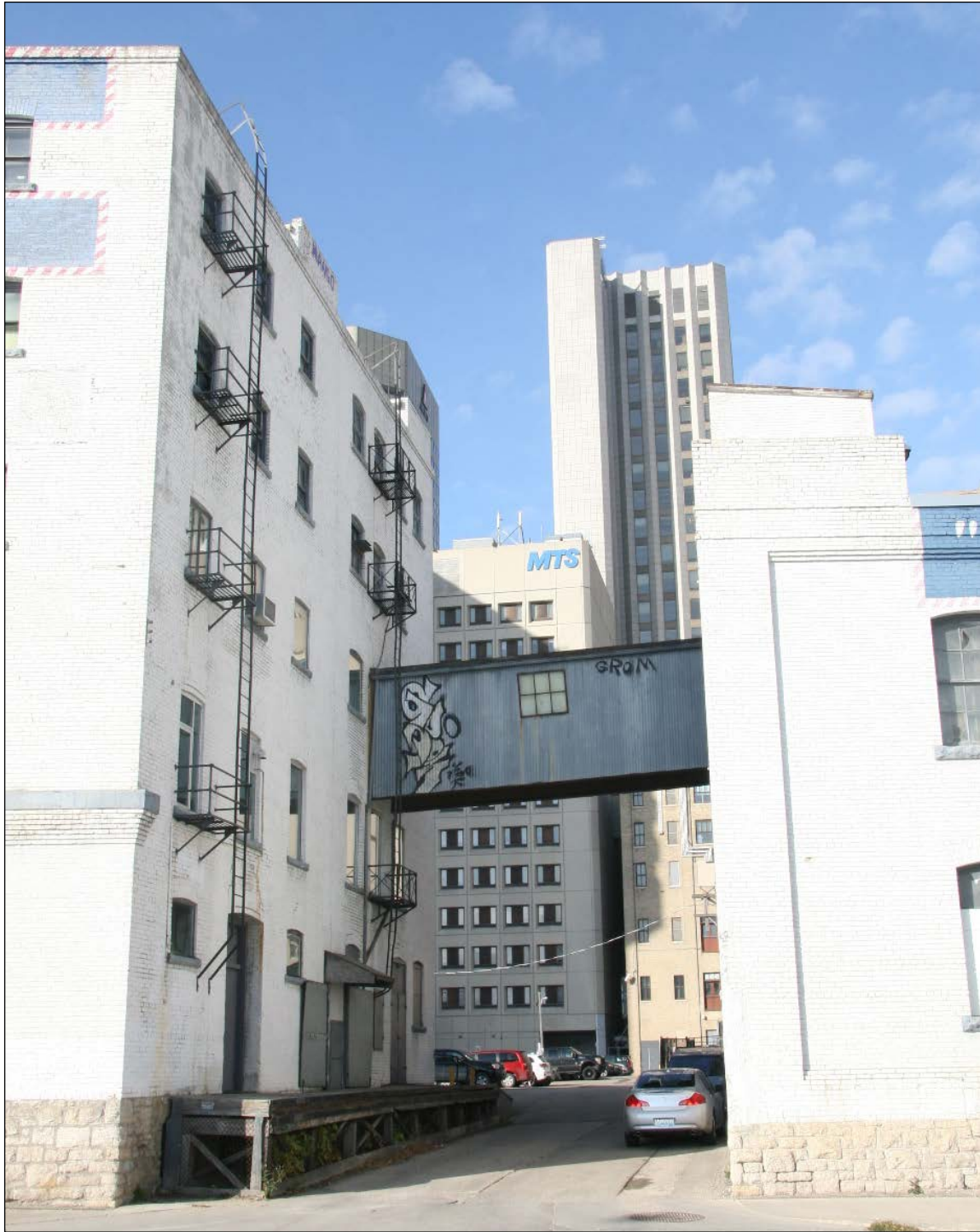
Plate 10 – Scott-Bathgate Building, 149 Pioneer Avenue, rear (north) façade, 2015. ( M. Peterson, 2015. )
