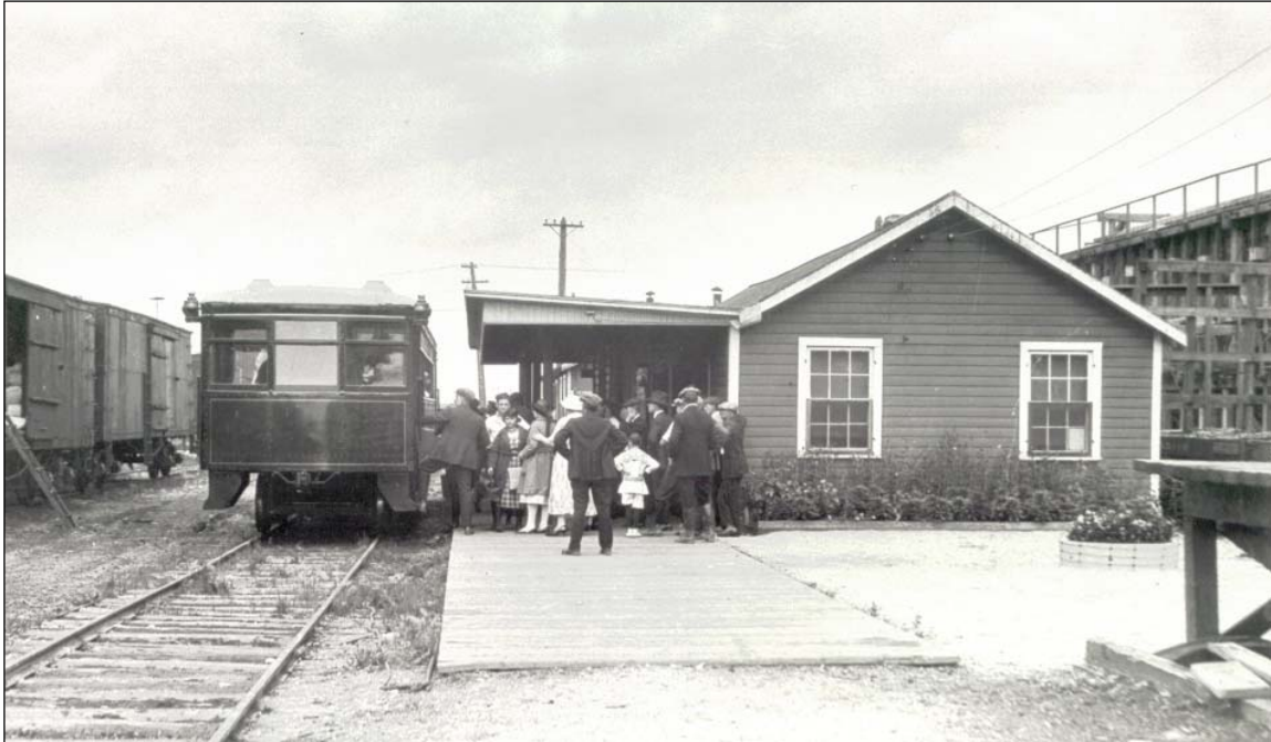
Plate 1 – Original Greater Winnipeg Water District Railway station, 598 Plinguet Street, ca.1923. (Courtesy of Western Canada Pictorial Index , Negative 513-16364.)
