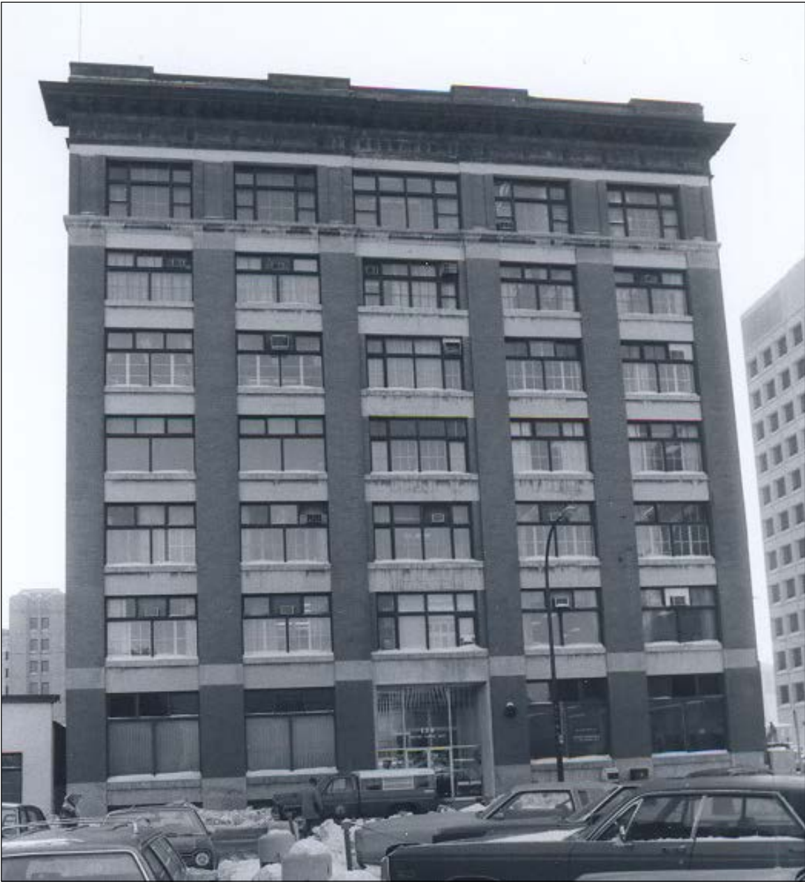
Plate 17 – Keewayden Block, 138 Portage Avenue, front (north) façade, 1978, showing the glazed transom windows. ( City of Winnipeg. )
