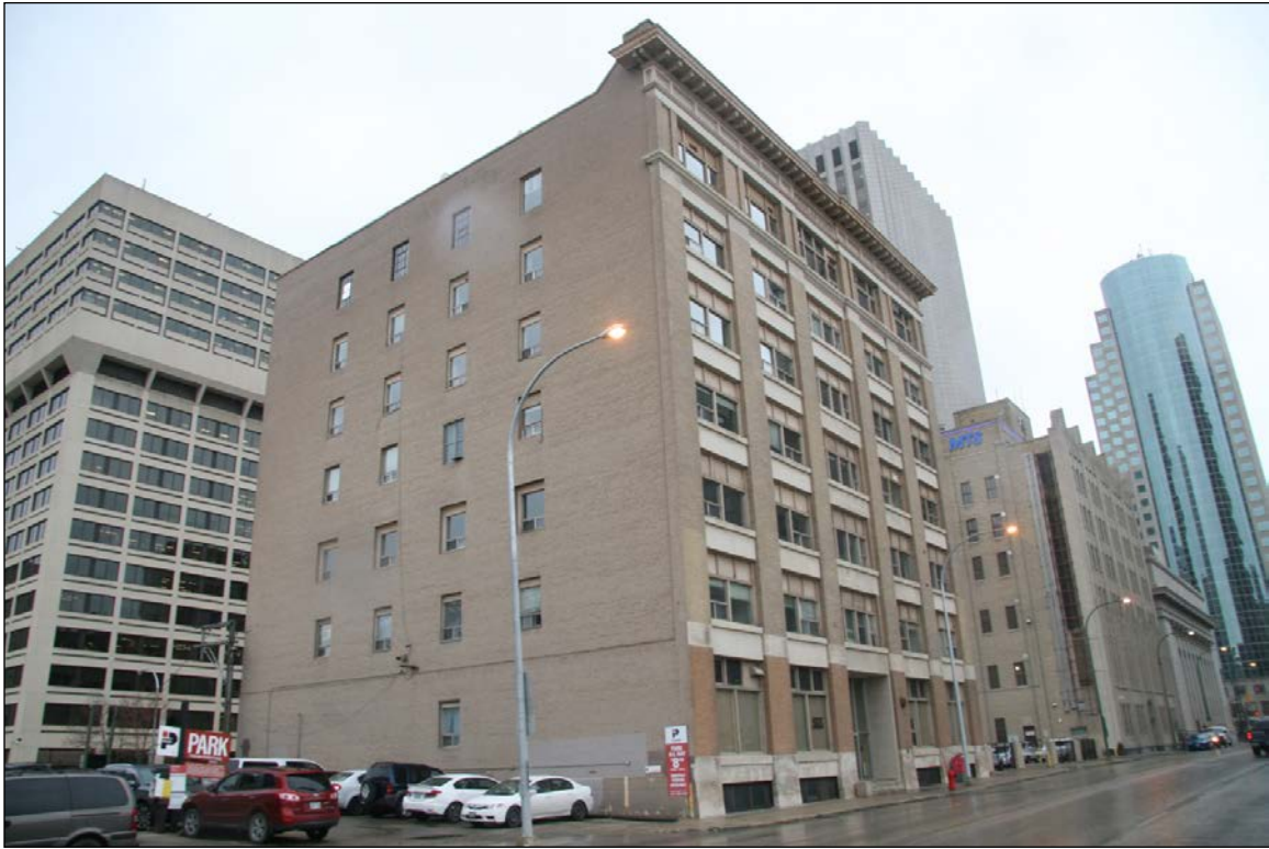
Plate 10 – Keewayden Block (Jacob-Crowley Building), 138 Portage Avenue, front & east façades, 2015 ( M. Peterson, 2015. )
