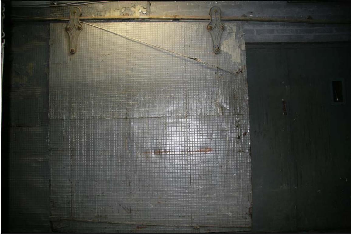
Plate 16 – Keewayden Block (Jacob-Crowley Building), 138 Portage Avenue, original basement fire door, 2016 ( M. Peterson, 2016. )
