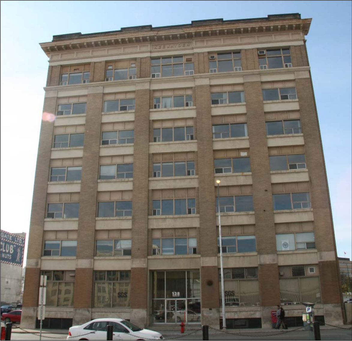
Plate 6 – Keewayden Block (Jacob-Crowley Building), 138 Portage Avenue, front (north) façade, 2015 (M. Peterson, 2015.)
