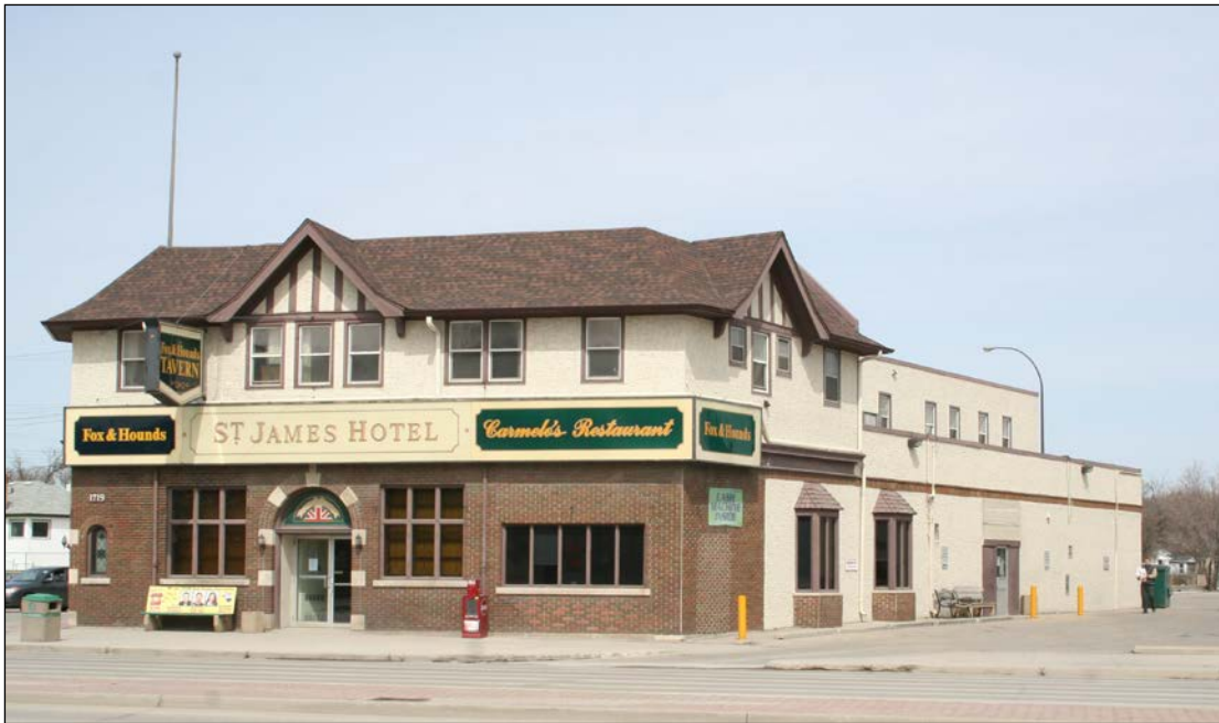
South and east façades, 2009
