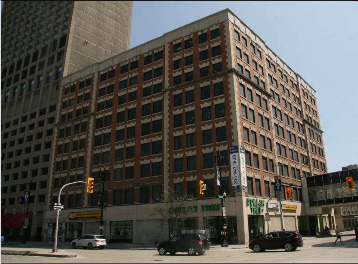
Plate 10 – Somerset Building, 294 Portage Avenue, north and west façades, 2019. ( M. Peterson, 2019. )
