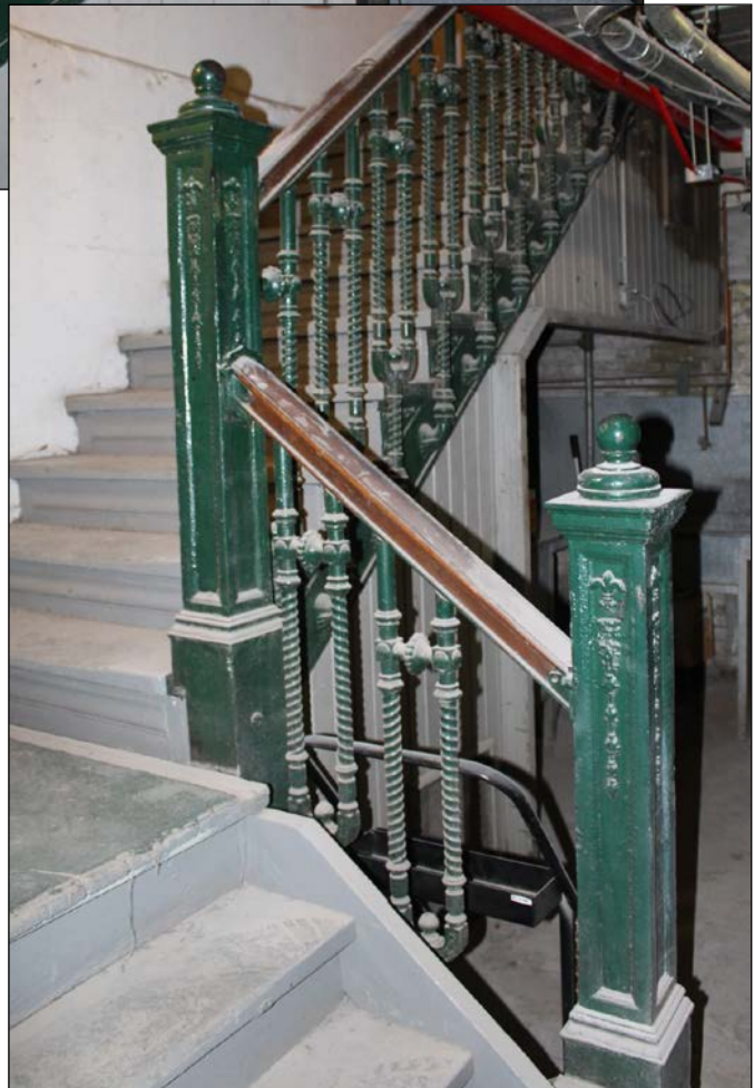
Plate 25 – Somerset Building, 294 Portage Avenue, basement stairs, 2019. (M. Peterson, 2019.)
