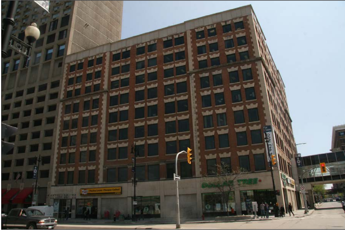
Plate 15 – Somerset Building, 294 Portage Avenue, front (north) and west façades, 2019. ( M. Peterson, 2019. )
