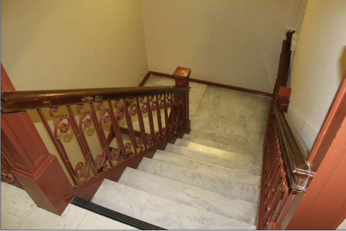
Plate 24 – Somerset Building, 294 Portage Avenue, southwest stairs, ninth floor, 2019. ( M. Peterson, 2019. )
