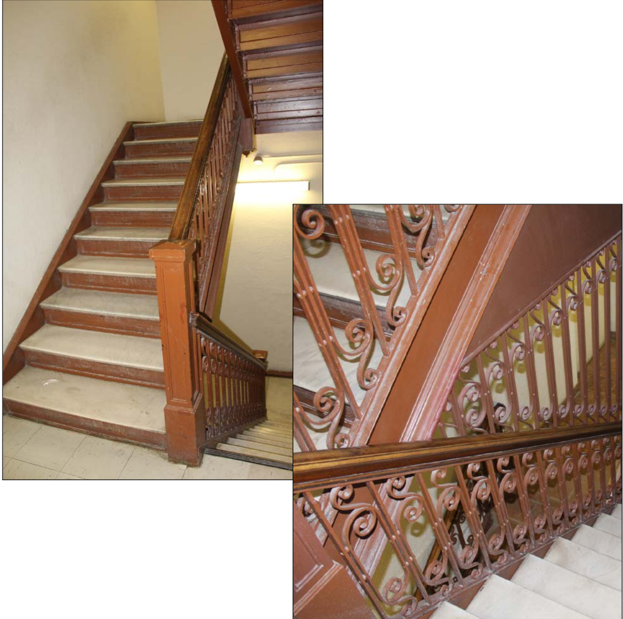
Plate 23 – Somerset Building, 294 Portage Avenue, east stairs, third floor, 2019. (M. Peterson, 2019. )
