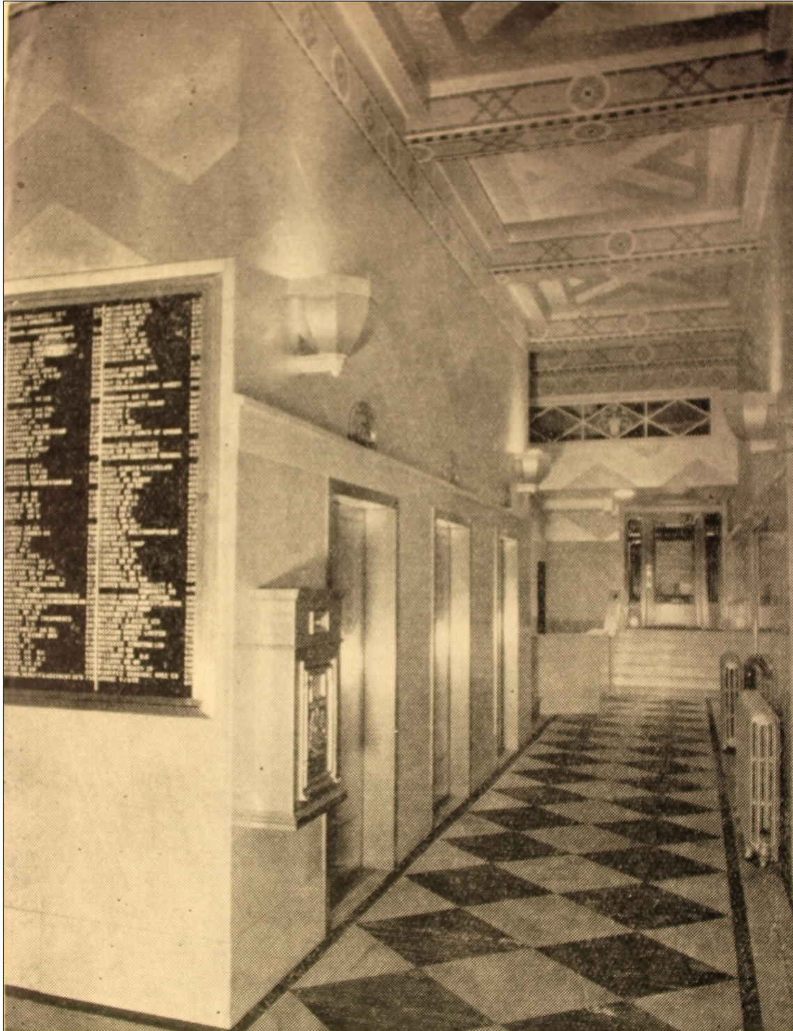
Plate 21 – Somerset Building, main lobby after 1935 alterations. (Reproduced from Western Canada Contractor and Builder , Nov.-Dec. 1935.)
