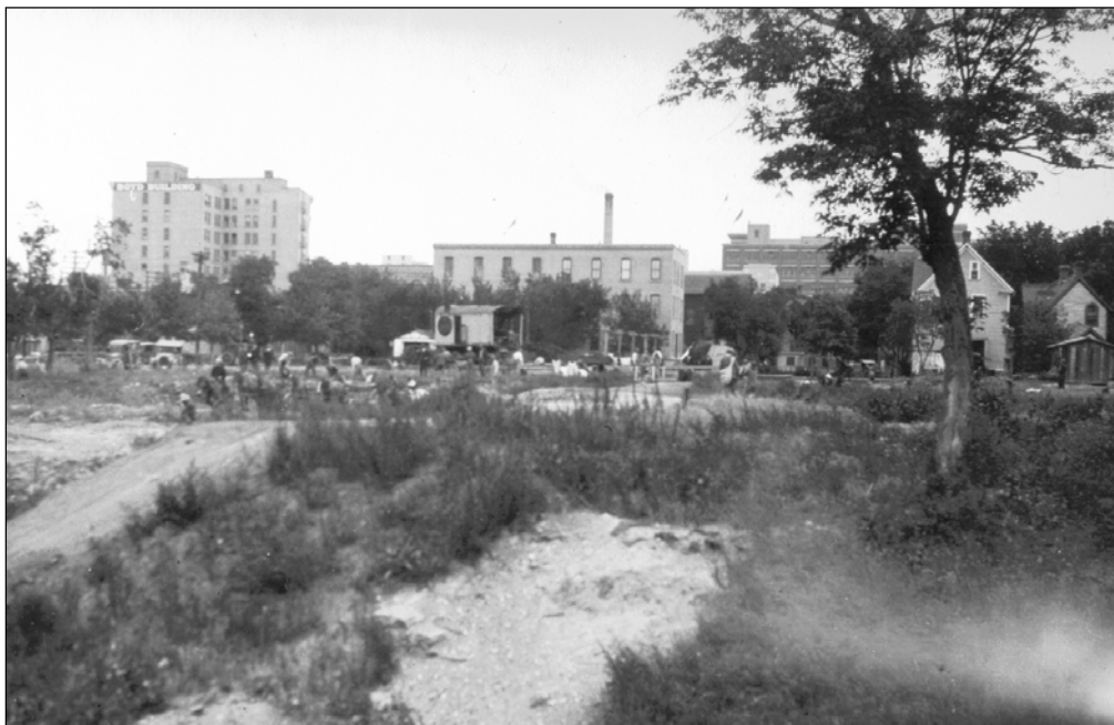
Plate 4 – When the foundations of the Hudson's Bay Company store were dug in 1925, the Boyd Building was very prominent for traffic coming eastward into the city centre. (Courtesy of the Provincial Archives of Manitoba, Thomas Burns Collection #152.)
