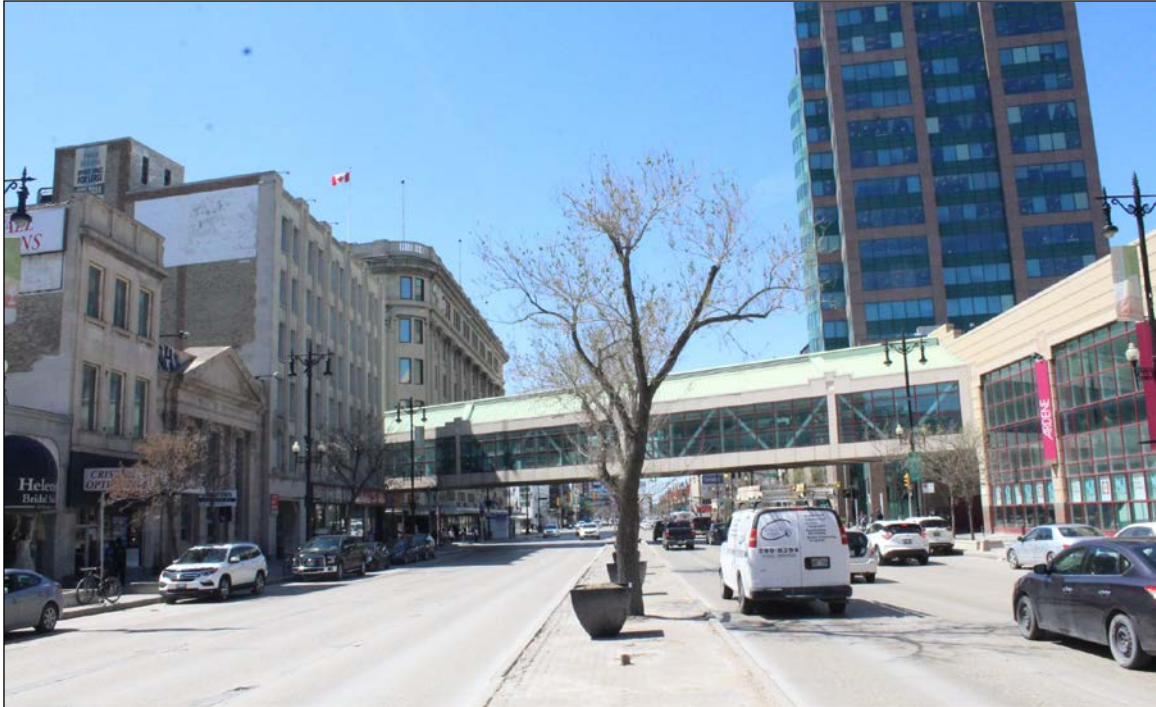
Plate 18 – Portage Avenue, looking west from Kennedy Street, 2019. (M. Peterson, 2019.)
