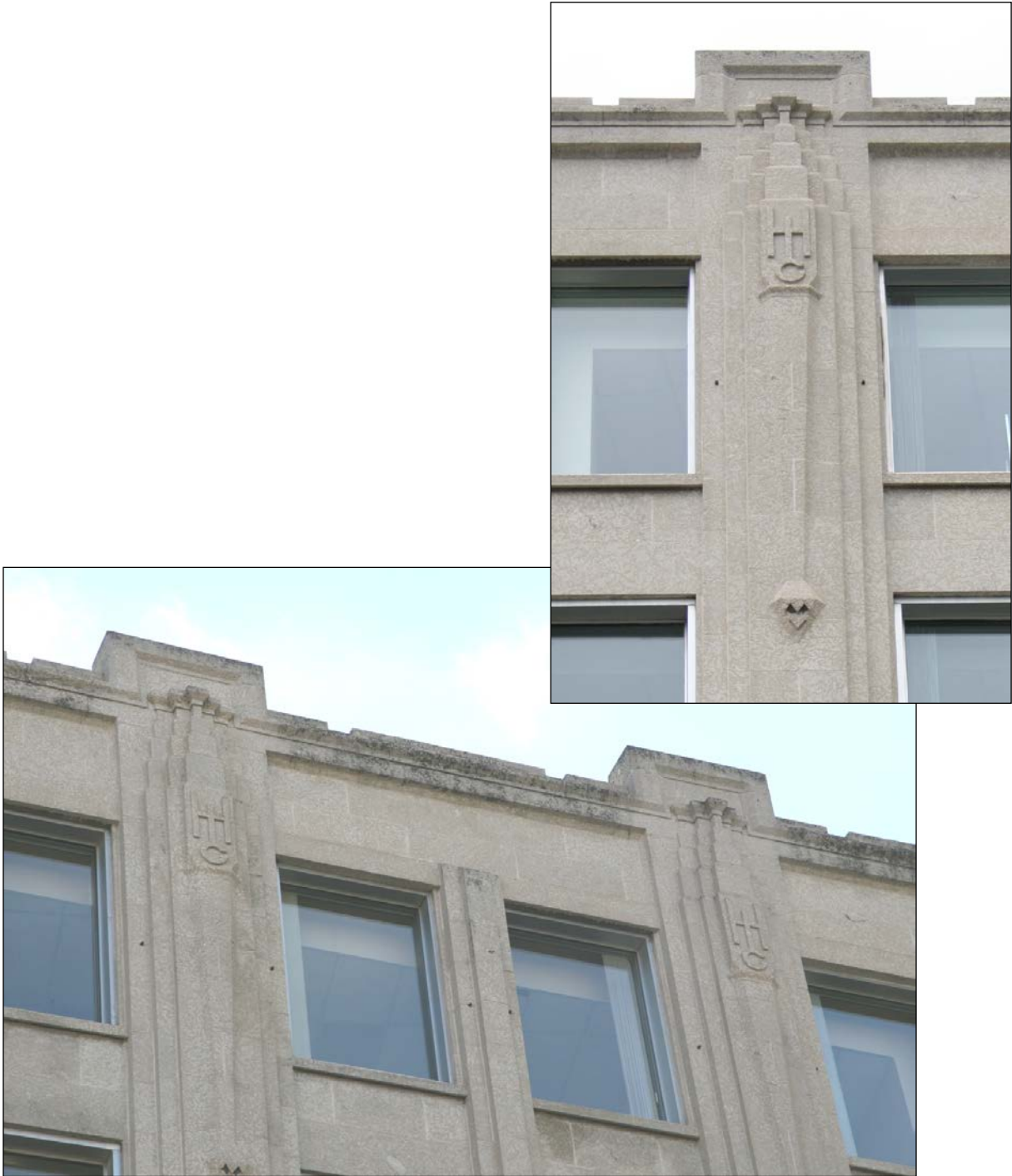
Plate 12 – Power Building, 428 Portage Avenue, detail of front (north) façade, 2015. ( M. Peterson, 2015. )
