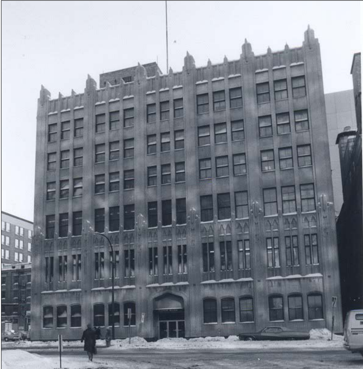
Plate 7 – Manitoba Telephones Building, 166 Portage Avenue, 1978. ( City of Winnipeg. )
