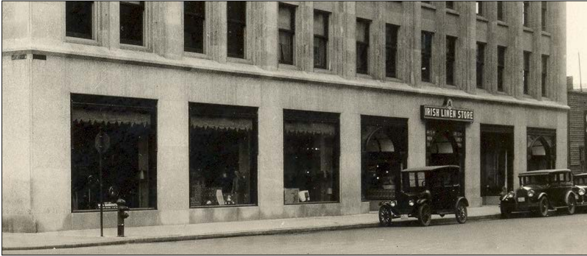
Plate 13 – Detail of the west side of the Power Building, shortly after construction in 1928. ( M. Peterson Collection. )
