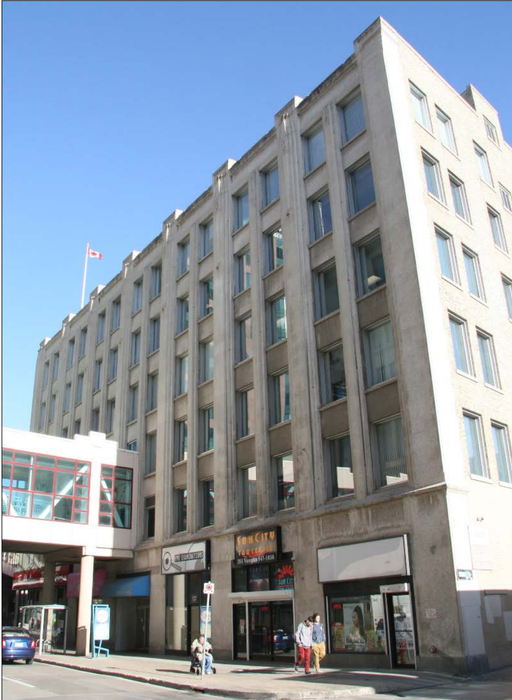
Plate 14 – Power Building, 428 Portage Avenue, west façade, 2015. (M. Peterson, 2015.)
