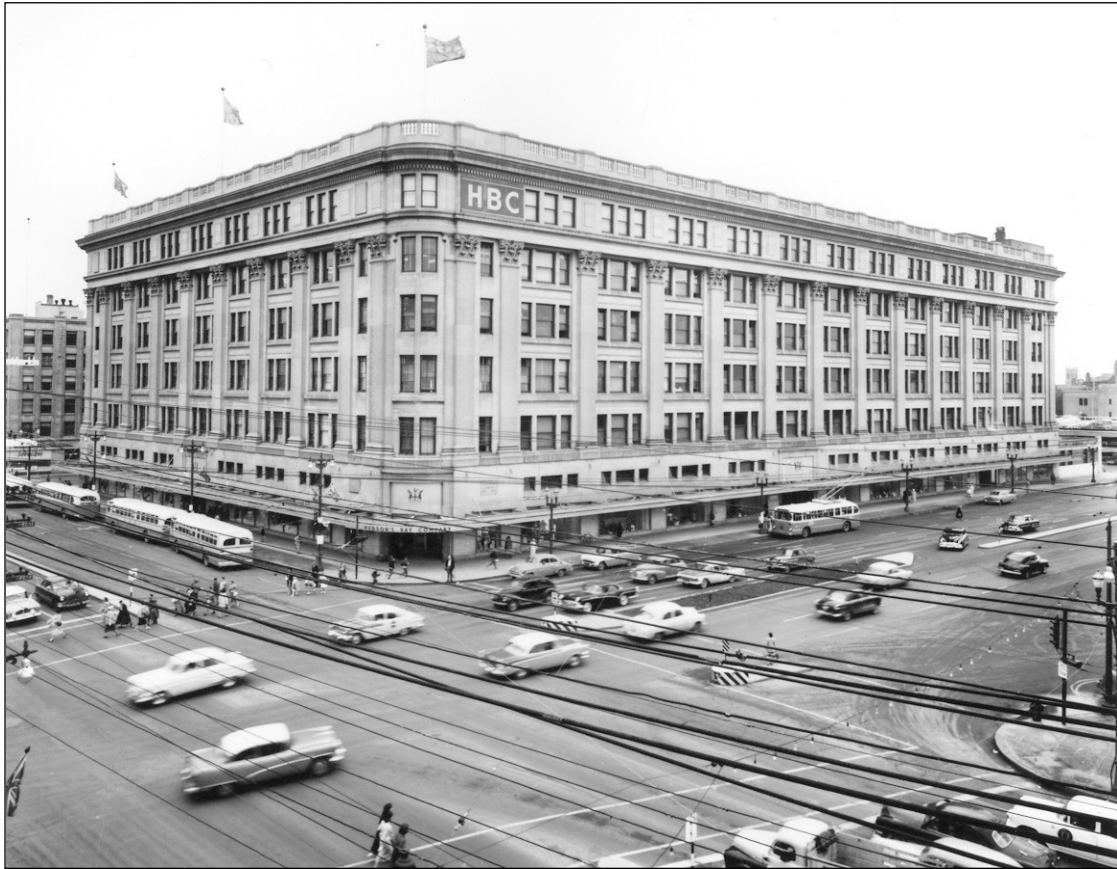
PLATE 46 - Hudson's Bay Company Store, 450 Portage Avenue, Winnipeg, 1957. In 1956, Moody and Moore designed the three-sided metal canopy which still encircles the Bay store. ( Hudson's Bay Company Archives )
