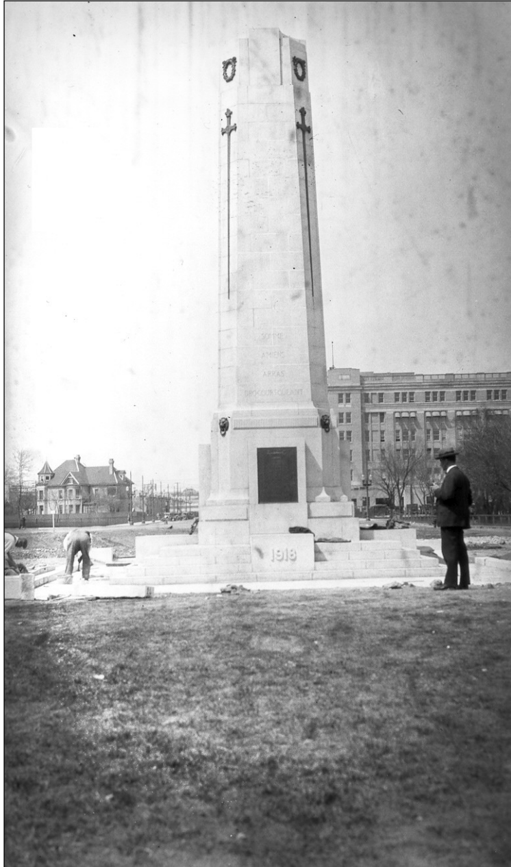
PLATE 54 - Cenotaph, Memorial Boulevard and York Avenue, 1929, Gilbert Parfitt, architect. Even a small structure such as this could be executed in limestone like the HBC Store in the background. ( Manitoba Archives )
