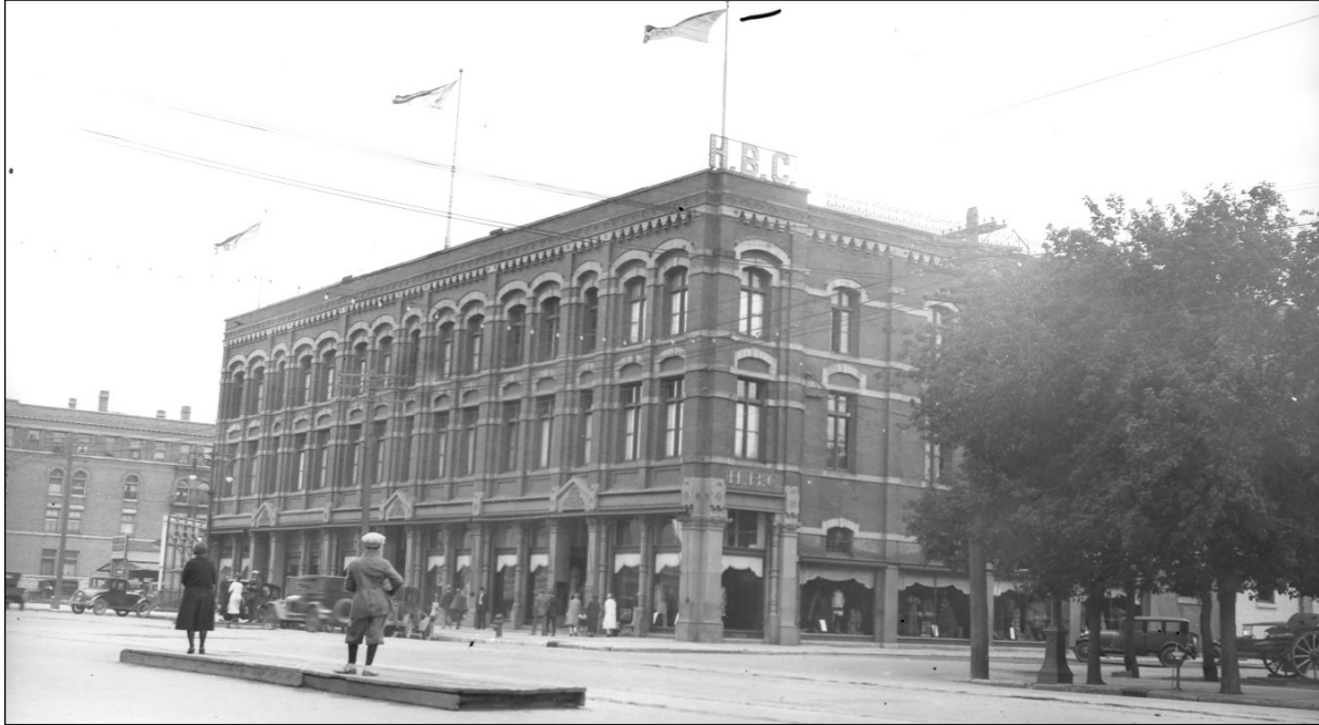
PLATE 1 - Hudson's Bay Company Store, 184 Main Street (SW – York Avenue), 1926. Designed by architect Balston C. Kenway in 1880-1881, and enlarged by George Browne in 1895 and 1899, this view shows the Main Street store some time during its final year of operation. ( Manitoba Archives )
