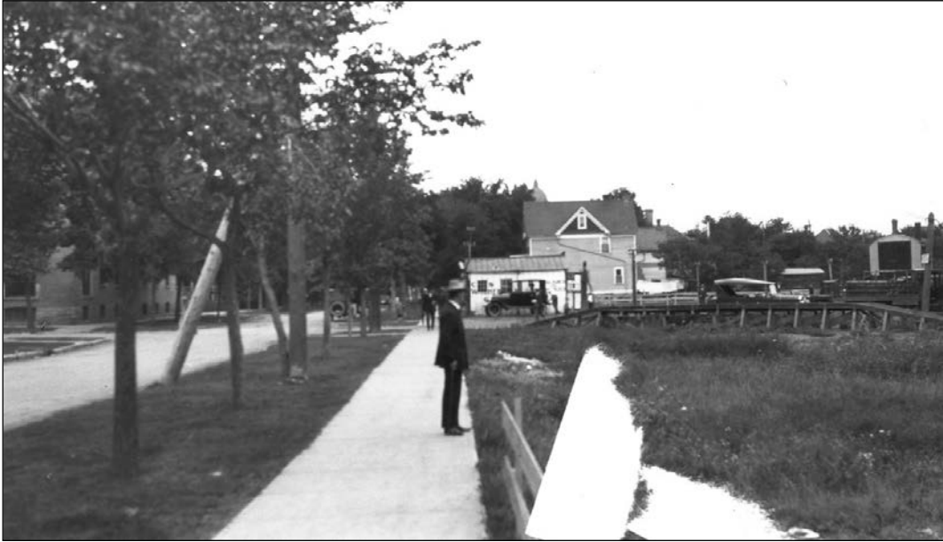
PLATE 24 - West Side, Vaughan Street, Looking South From Portage Avenue, September 1925. This peaceful, tranquil scene was about to be disturbed by the construction of the new HBC Store. ( Manitoba Archives )
