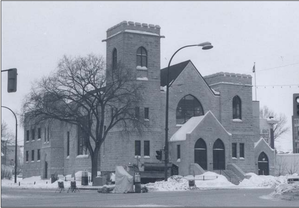
Front (north) and east façades, 1978
