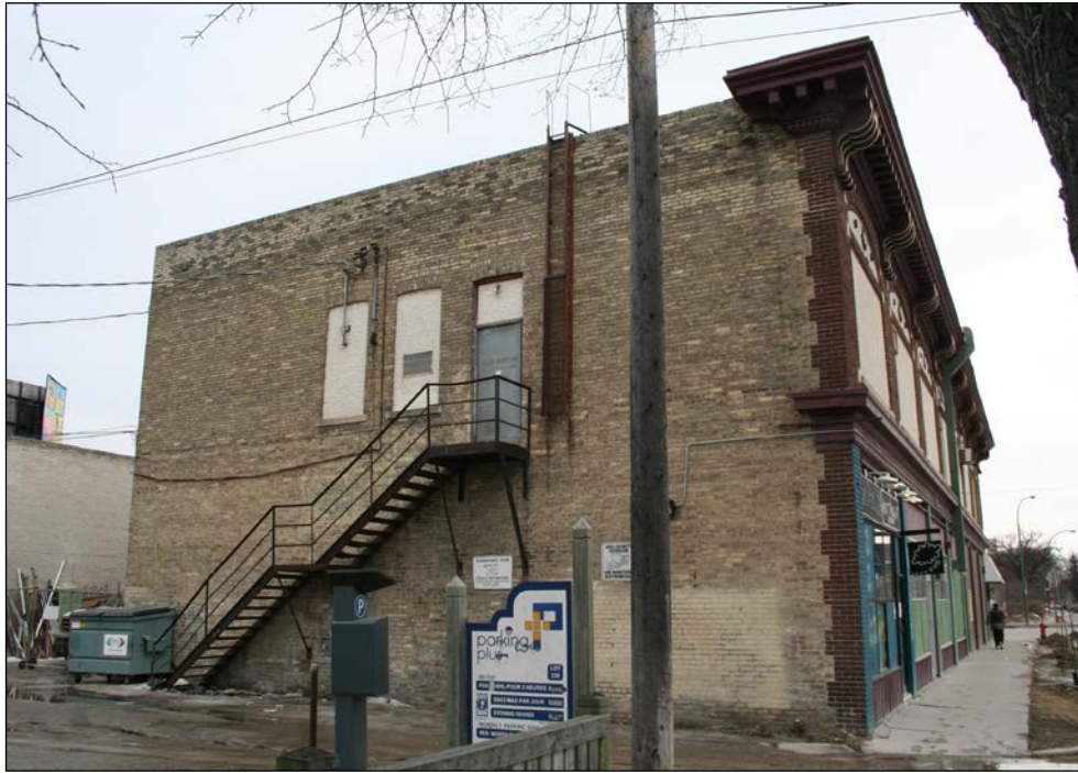
Rear (north) and west façades, 2008
