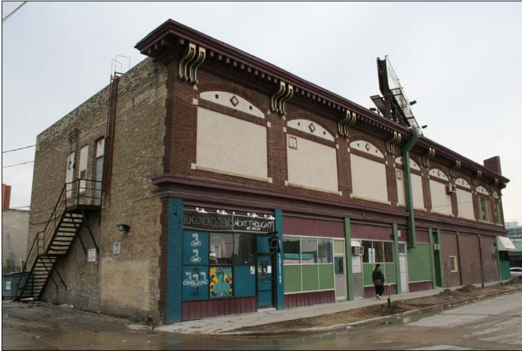
Rear (north) and west façades, 2008
