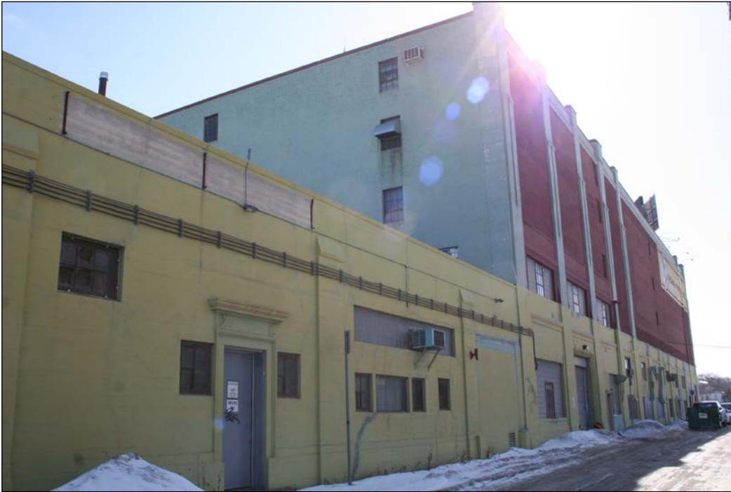
Rear (north) and west façade, 2008
