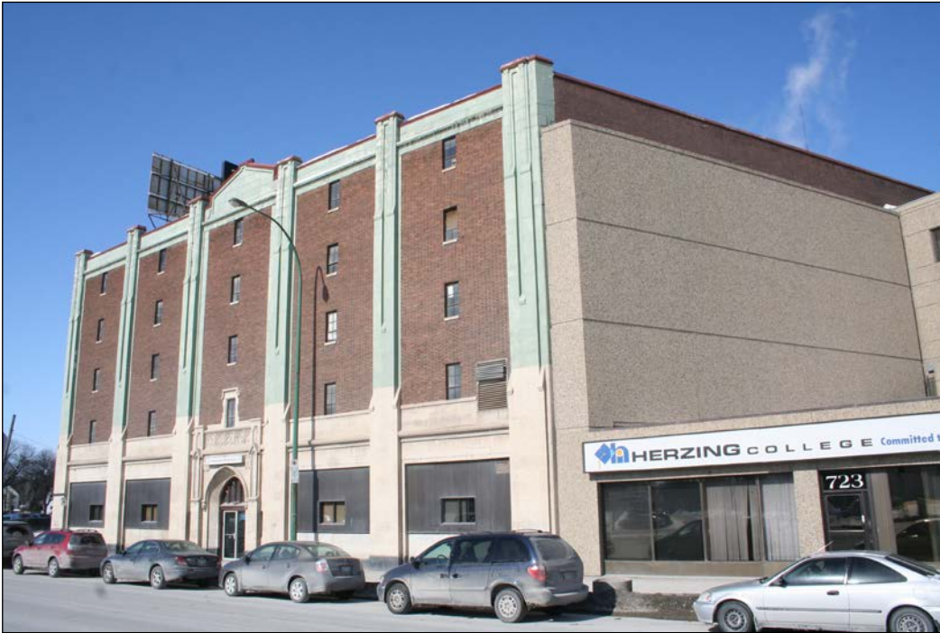
Front (south) and east façades, 2008
