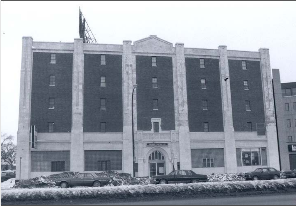
Front (south) façade, 1978
