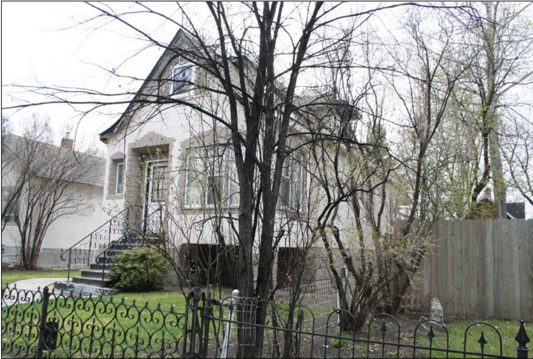
Front (east) and north façades, 2009
