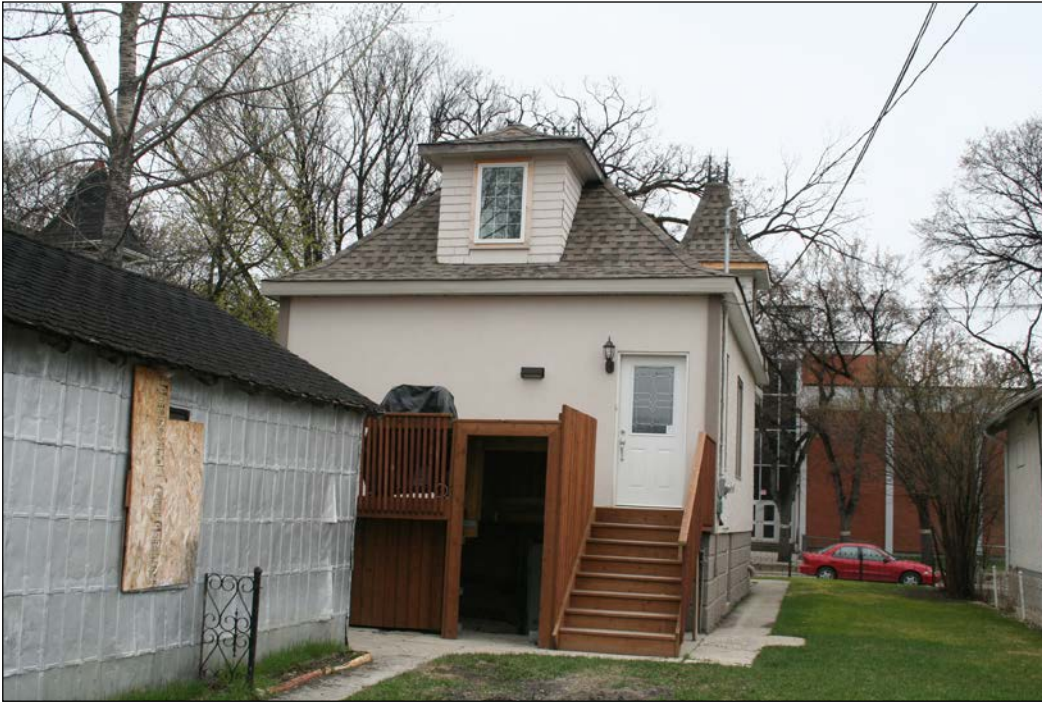
Rear (west) and south façades, 2009
