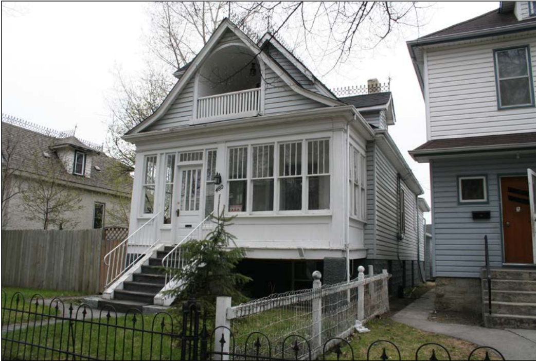
Front (east) and north façades, 2009
