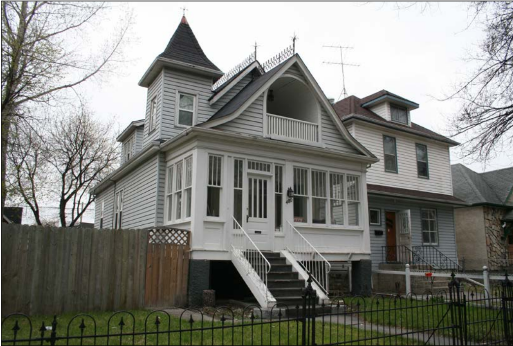
Front (east) and south façades, 2009
