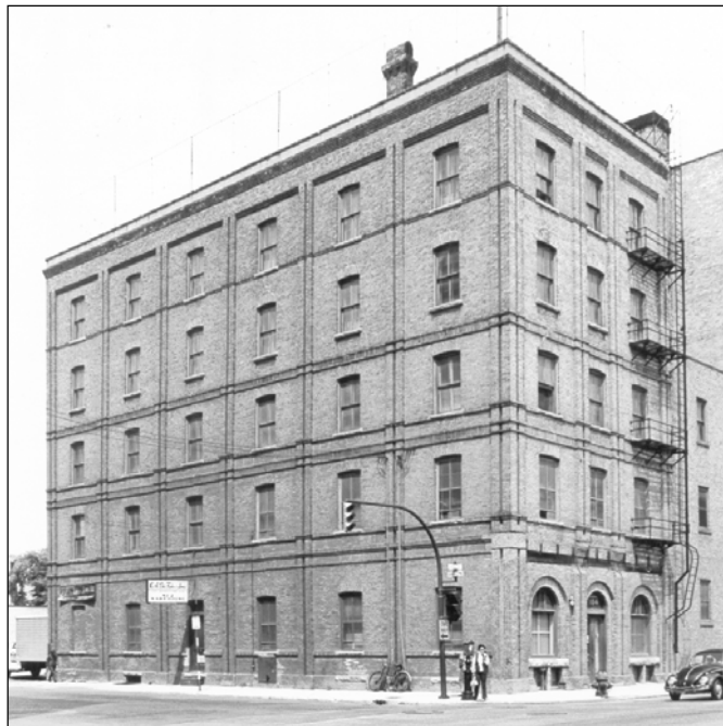
Plate 4 – 104-108 Princess Street, 1970. . ( Courtesy of the Provincial Archives of Manitoba, Architectural Survey. )
