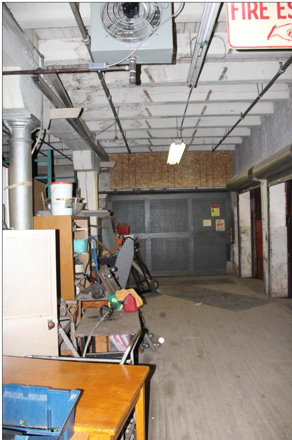
Plate 16 – Cockshutt Plow Company Building, 238 Princess Street, main floor shipping and receiving area with freight elevators, 2019. ( M. Peterson, 2019. )
