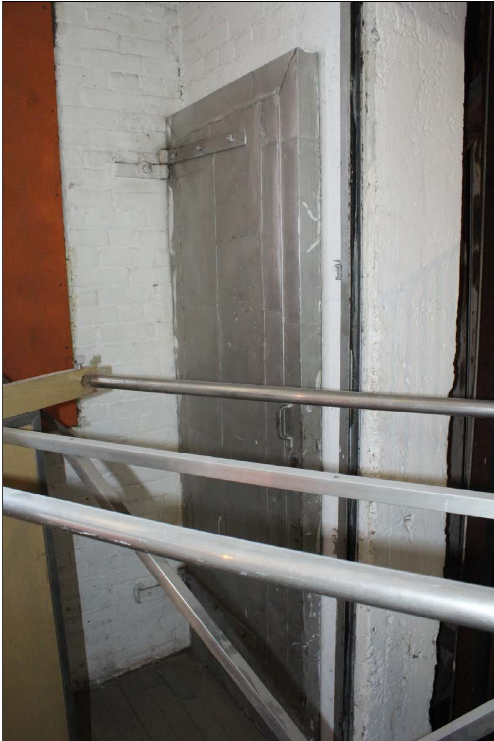
Plate 18 – Cockshutt Plow Company Building, 238 Princess Street, metal clad fire door, elevator shaft staircase, third floor, 2019. (M. Peterson, 2019.)
