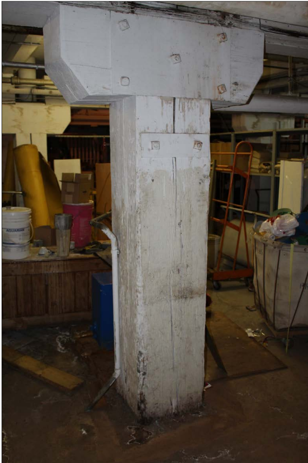
Plate 13 – Cockshutt Plow Company Building, 238 Princess Street, basement post, 2019. ( M. Peterson, 2019. )
