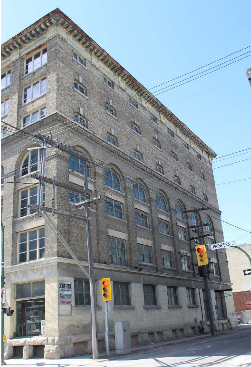
Plate 9 – Cockshutt Plow Company Building, 238 Princess Street, north façade, 2019. ( M. Peterson, 2019. )
