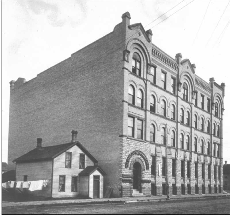
Plate 1 – The Peck Building, 33 Princess Street, ca.1896. (Courtesy of the Provincial Archives of Manitoba, Gisli Goodman Collection #1 [N7119].)
