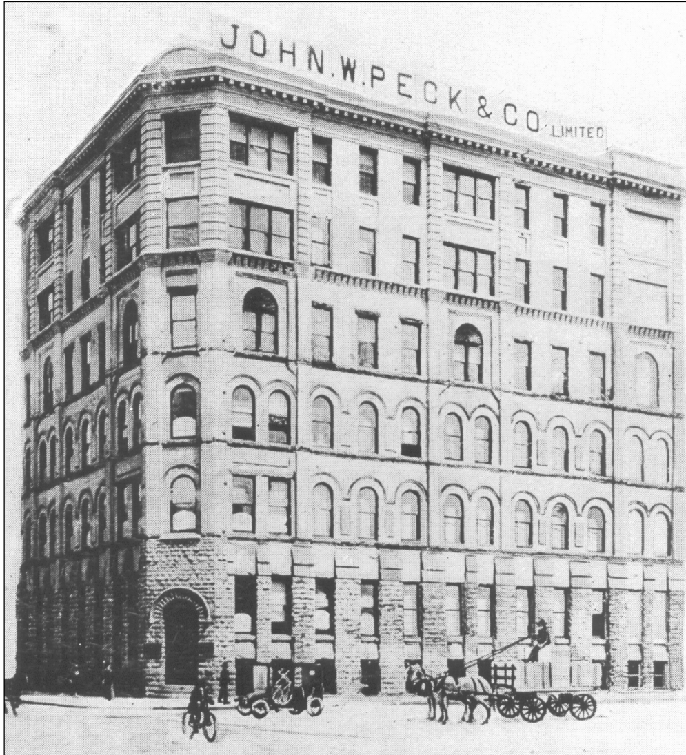
Plate 3 – The Peck Building with its addition, 1907. ( Courtesy of the Provincial Archives of Manitoba, N7104. )
