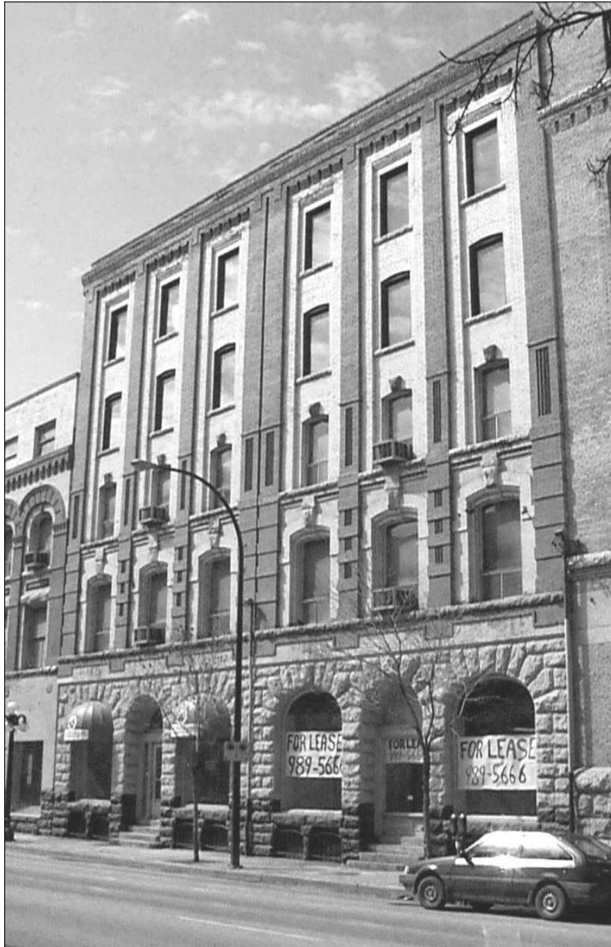
Plate 6 – 78 (86-88) Princess Street, front (east) façade. (M. Peterson, 1998.)
