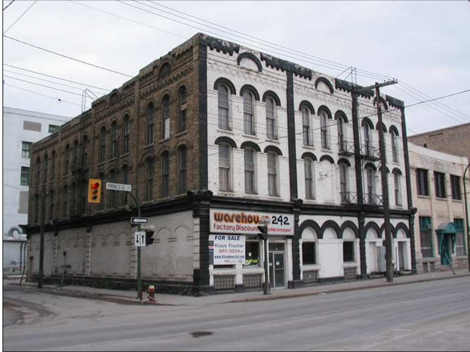
Plate 8 – Bathgate Block, front (east) and south façades, 2002. ( M. Peterson, 2002. )
