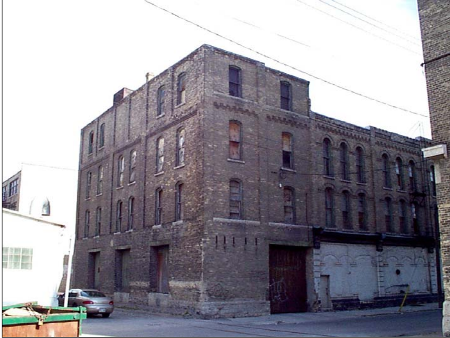
Plate 3 – Rear addition of the Bathgate Block, prior to demolition. (M. Peterson, 2000.)
