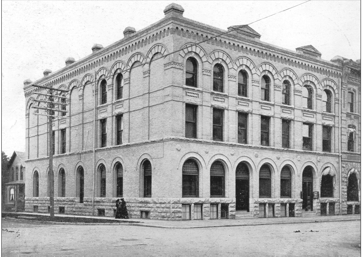
Plate 3 – Kenneth Mackenzie Co. warehouse, 78 Princess Street, ca.1903. ( M. Peterson Collection. )
