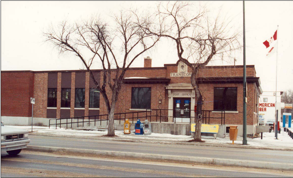
Front (south) façade, no date
