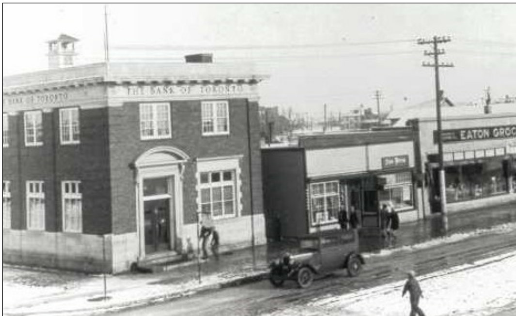
Plate 2 – Bank of Toronto, 1935. (Courtesy of the Provincial Archives of Manitoba, Frank Munton Collection, N19704.)
