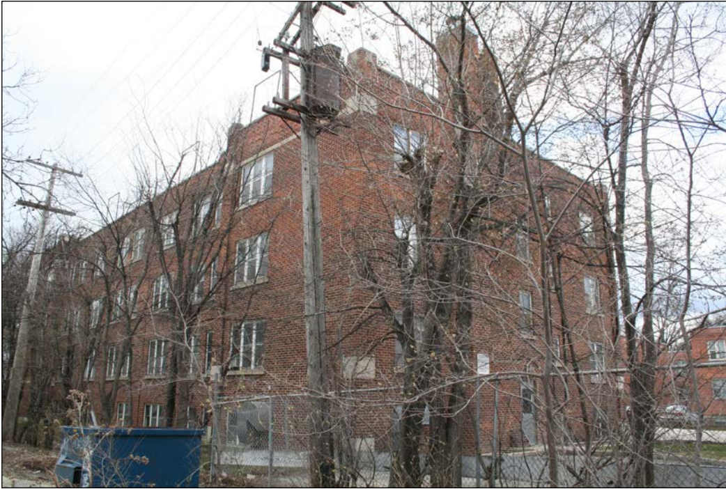
Rear (north) and east façades, 2009
