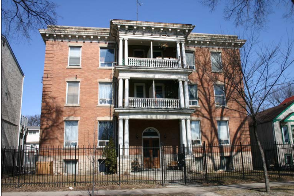
Plate 1 – 141 River Avenue, Ludlow Court Apartments, front (south) façade, 2005. (M. Peterson, 2005.)
