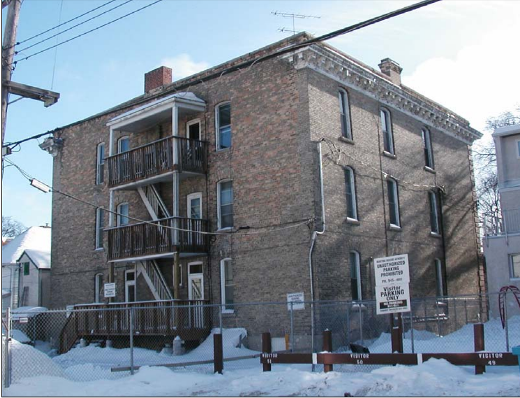
Plate 3 – Rear (north) and west side, 2005. ( M. Peterson, 2005. )
