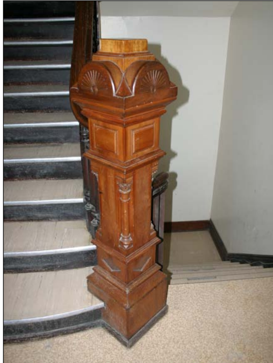
Plate 9 – Newel post of main staircase, ground floor, 2005. ( M. Peterson, 2005. )
