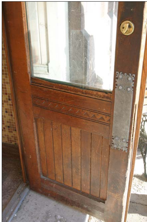
Plate 8 – Detail of main (south) door, 2005. (M. Peterson, 2005.)
