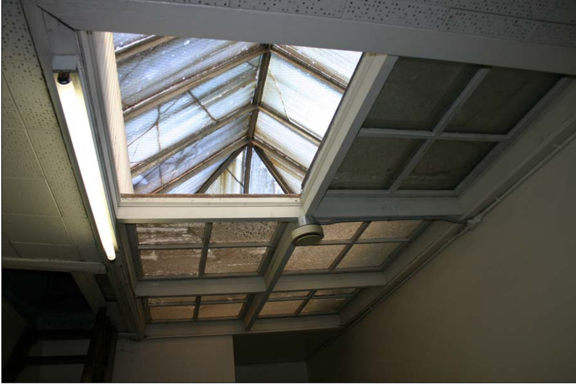
Plate 12 – Staircase skylight, 2005. ( M. Peterson, 2005. )
